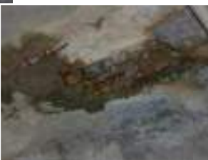
Spalling and penetrating cracks in concrete overlay
