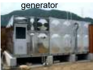
Potable water storage tank
