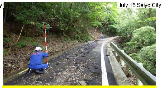
Survey of roads in which large cracks have appeared due to heavy rain
