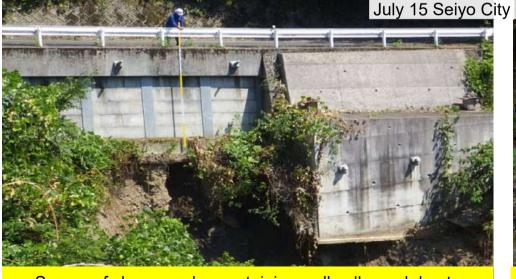
Survey of slopes under a retaining wall collapsed due to heavy rain
