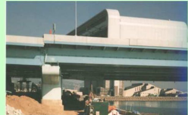
Warped pier foundation due to fluidization (Great Hanshin Earthquake)
