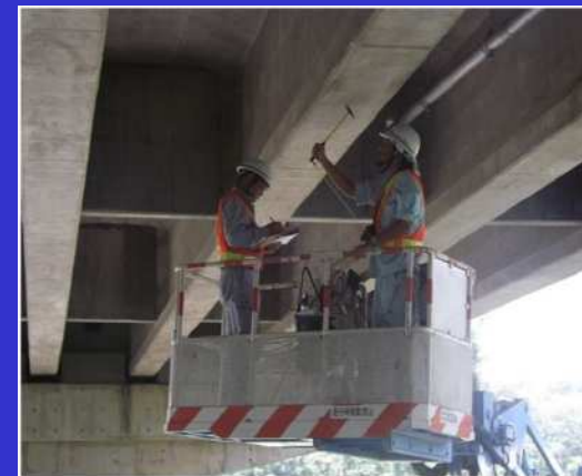
Ensuring soundness with close-up visual inspections
