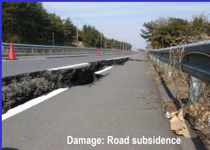
Damage: Cracked road
