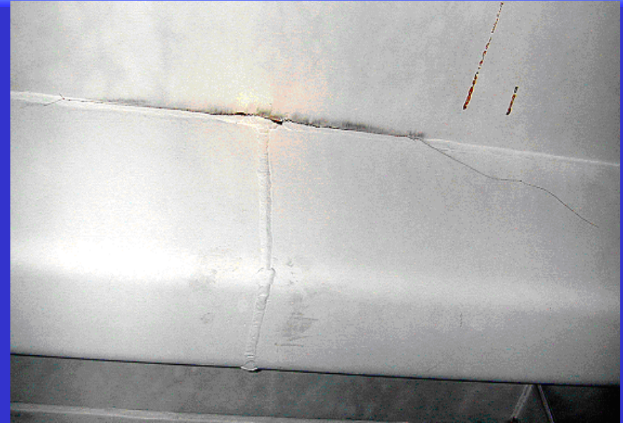
Steel plate deck: Longitudinal rib and deck plate joint
