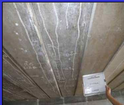
Cracks in the main girder due to salt damage
