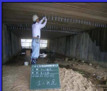
Filling cracks
