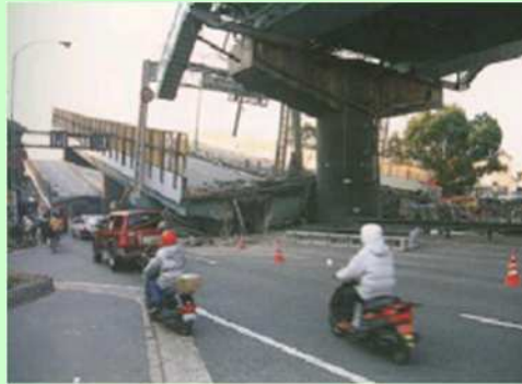
Collapse of elevated simple girder bridge (Great Hanshin Earthquake)
