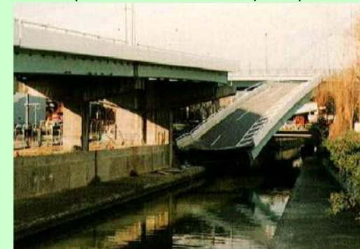
Collapse of curved bridge (Great Hanshin Earthquake)
