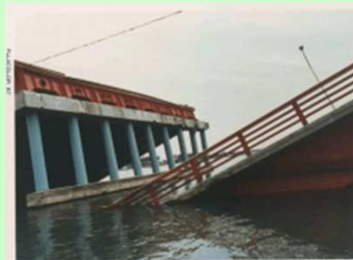
Collapse due to liquefaction/fluidization (Niigata Earthquake)
