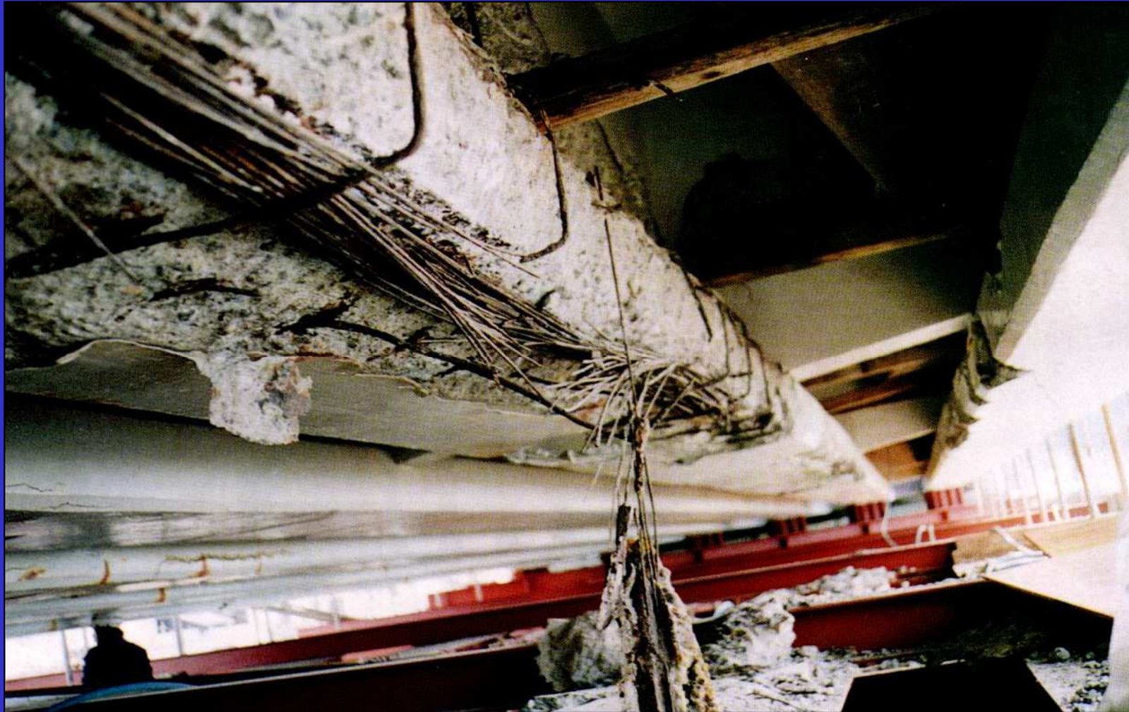
Snapped steel wires in an aging prestressed concrete bridge
