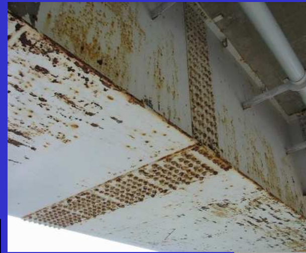
Deteriorated coatings
