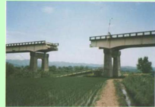
Collapse of cantilever girder bridge (2005 Miyagi Earthquake)
