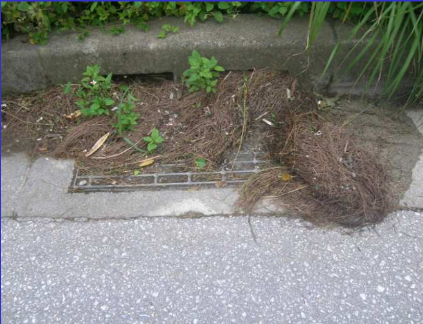
Drain clogged with leaves, dirt, and other debris
