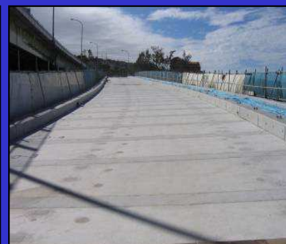
Concrete slab replaced
