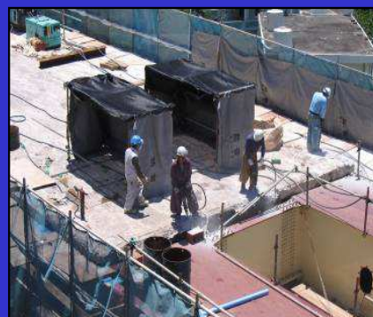
Removal of concrete slab
