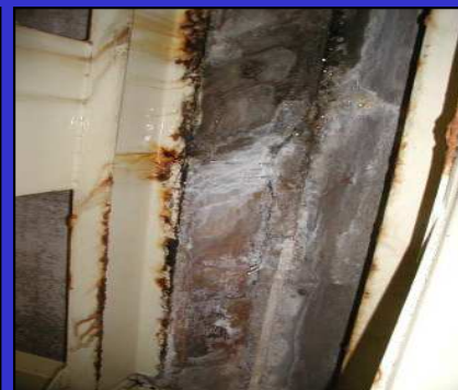
Cracks in the concrete due to salt damage with swelling as a result
