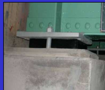
Girder ends reinforced with cover plates and coated, supports replaced
