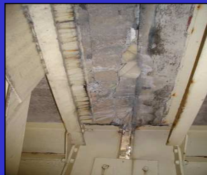
Cracks in the concrete due to salt damage with swelling as a result
