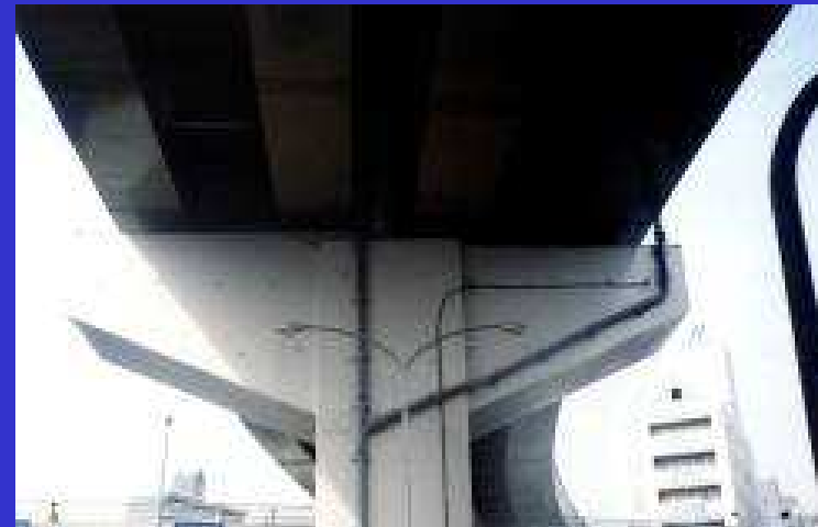
Steel plate bonding method
