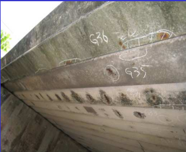
Concrete exfoliation (salt damage)
