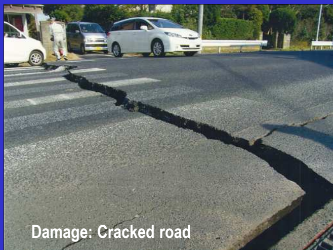
Damage: Road shift
