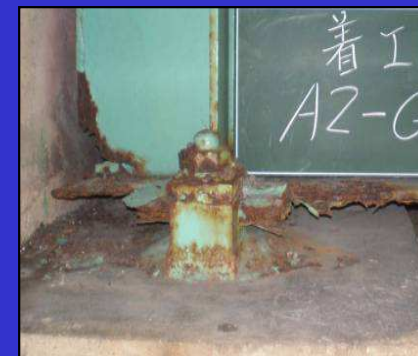
Salt corrosion at girder ends, damaging supports
