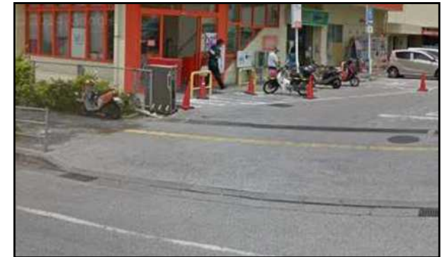
Lowering the sidewalk to allow boarding
