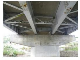
Steel corrosion caused by salt damage, lack of an anti-collapse system
