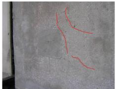
Cracking at the main girder ends caused by alkali-aggregate reaction
