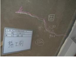
Cracks and delamination have occurred in the concrete deck due to salt damage.
