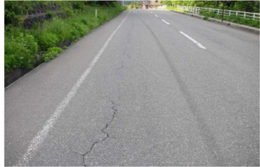
Linear crack
