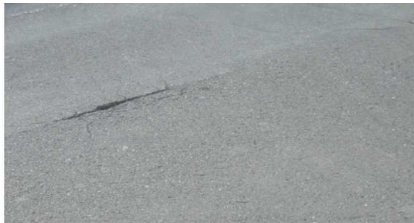
Construction joint cracks
