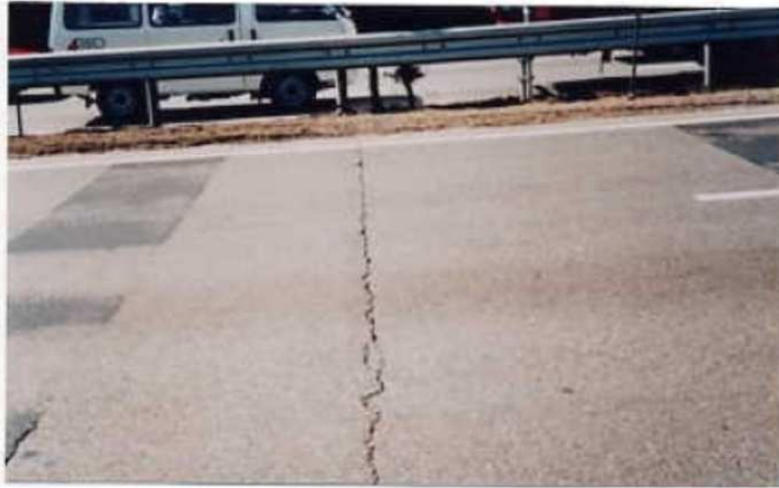
Reflection crack
