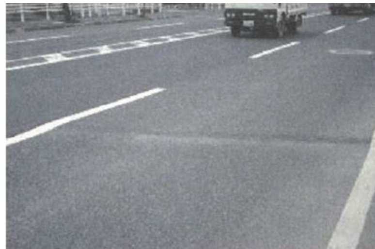
Linear crack
