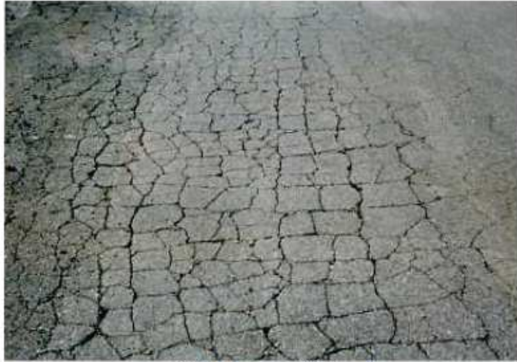
Mesh-like cracks
