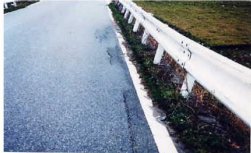
Cracks caused by displacement
