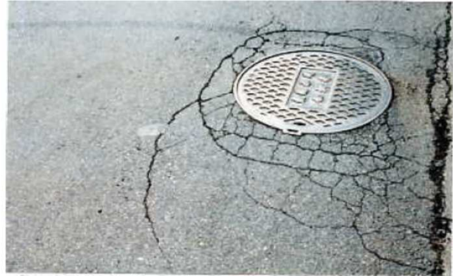
Cracks caused by structure
