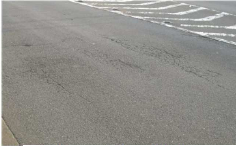
Cracking caused by subsidence
