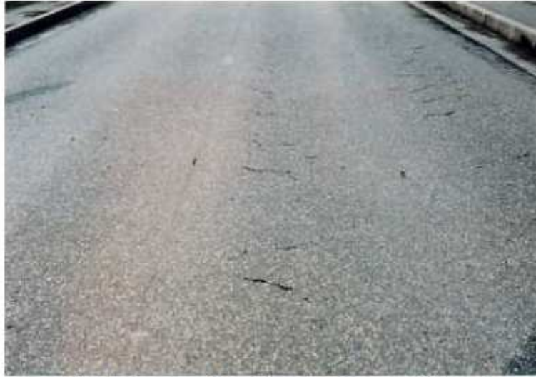
Cracks caused by surface displacement
