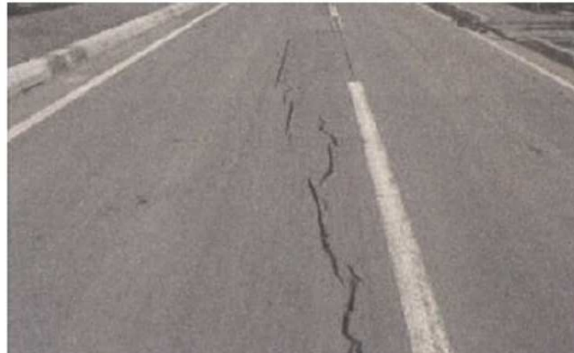
Cracks caused by freezing
