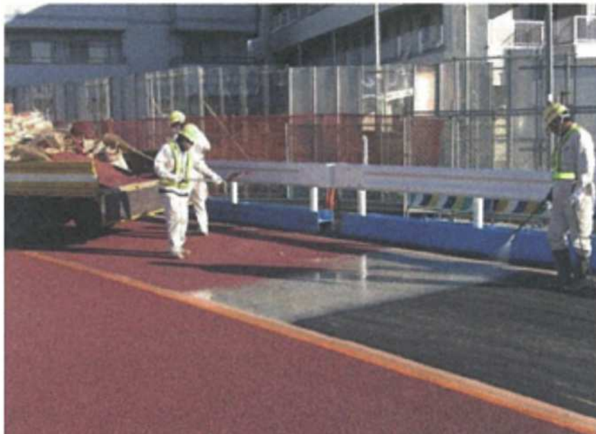
Coating of resin materials
