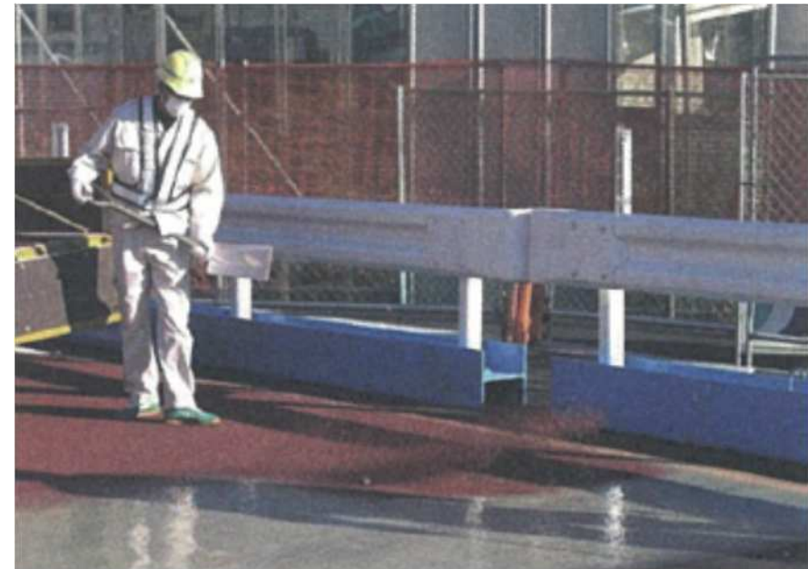
Spraying of aggregate
