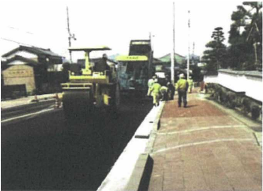
Cutting overlay method
