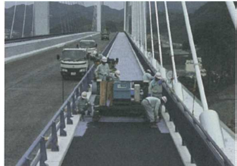
Construction of permeable resin mortar filling method
