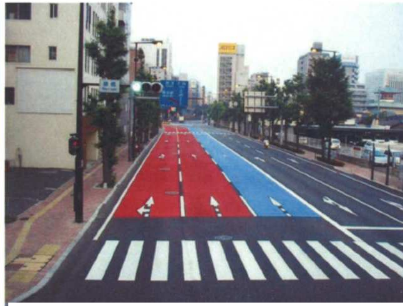
Photo 6 Lane guidance construction example
