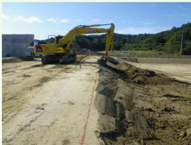
Liner construction with bentonite mixed soil
