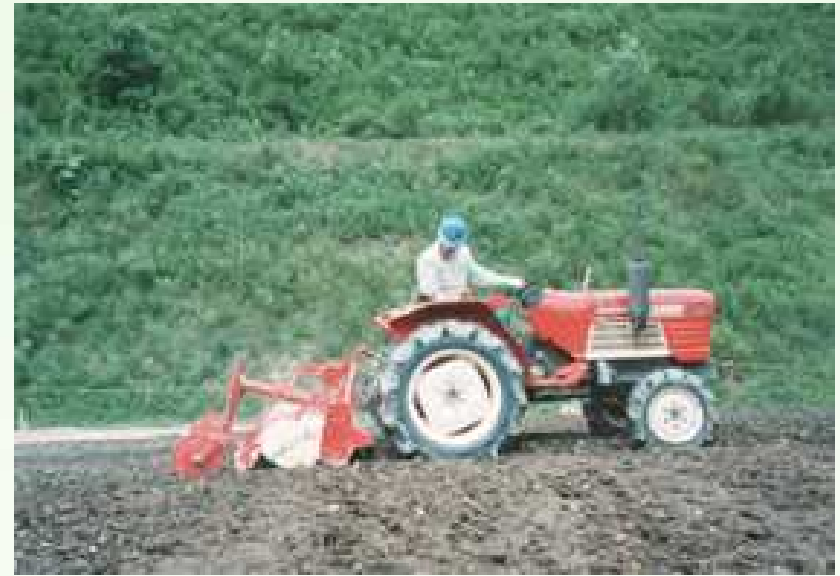
Modifier are added and mixed using tractor
