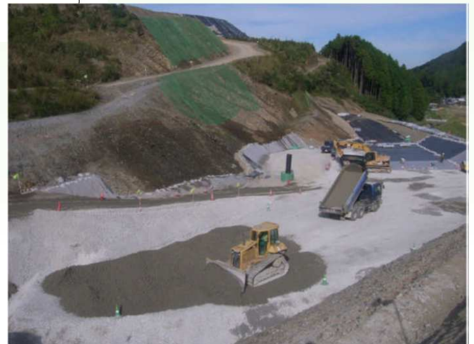
Embankment construction status with insoluble soil
