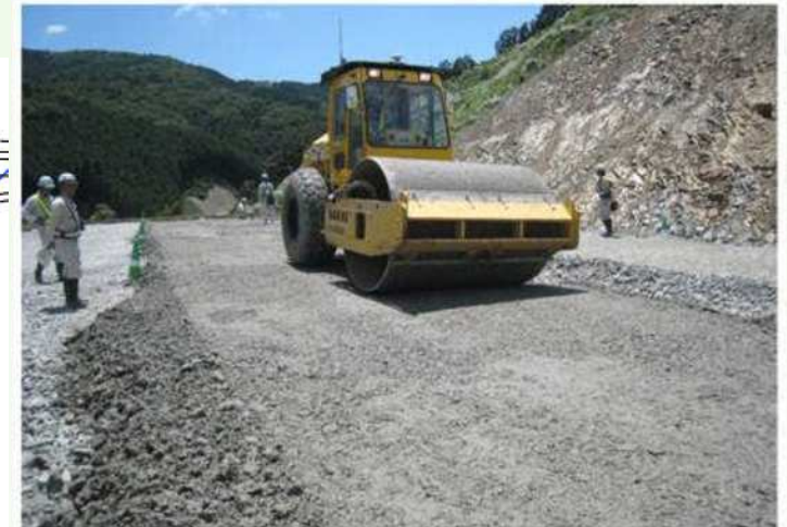
Insolubilization test using cement type solidifier
