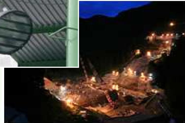
To prevent light diffusion by hood louvers and avoid death of insects by adopting less insect-inducing lamp
