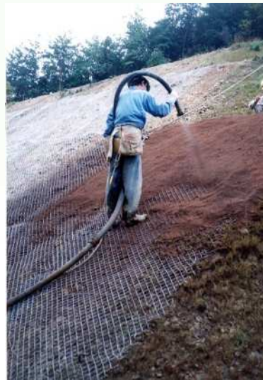
Sprayed by mixing with seeds, etc.
