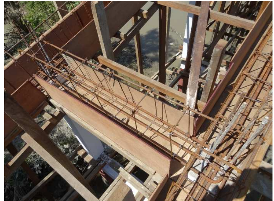
Form work for the beam
