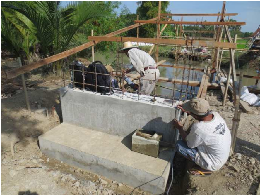
Assembling steel bar
