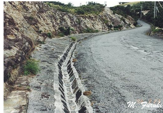
An inverted trapezoidal road gutter made before the restoration (near the Tokashiki Island Meteorological Observatory Station)
