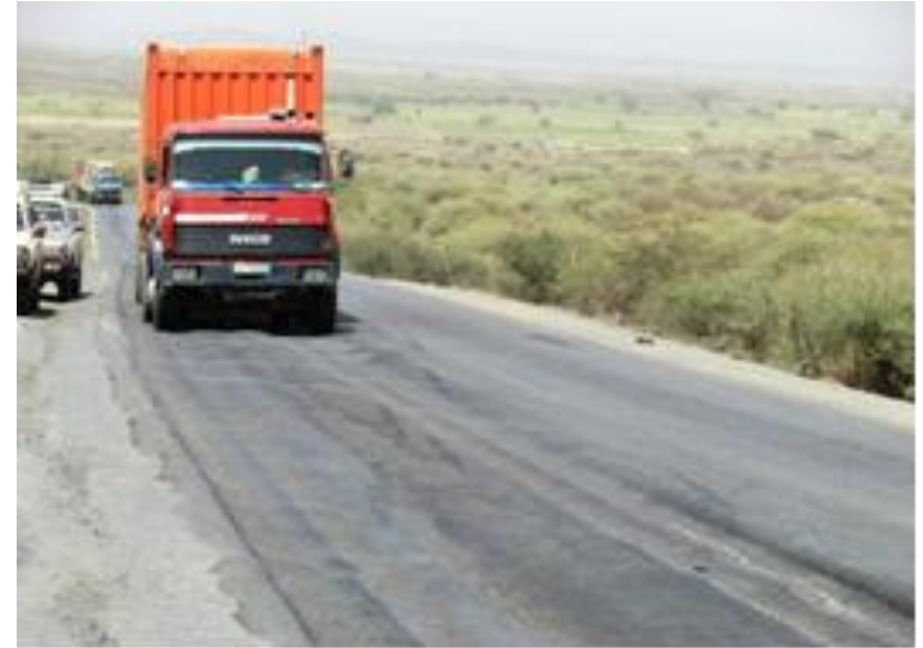
Fig. Deep rutting at a uphill section of road A1 in Ethiopia
