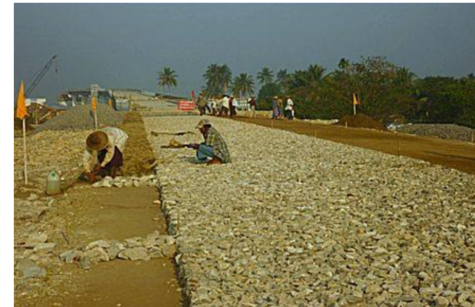
Fig. Shoulder cross drain(in Myanmar)
