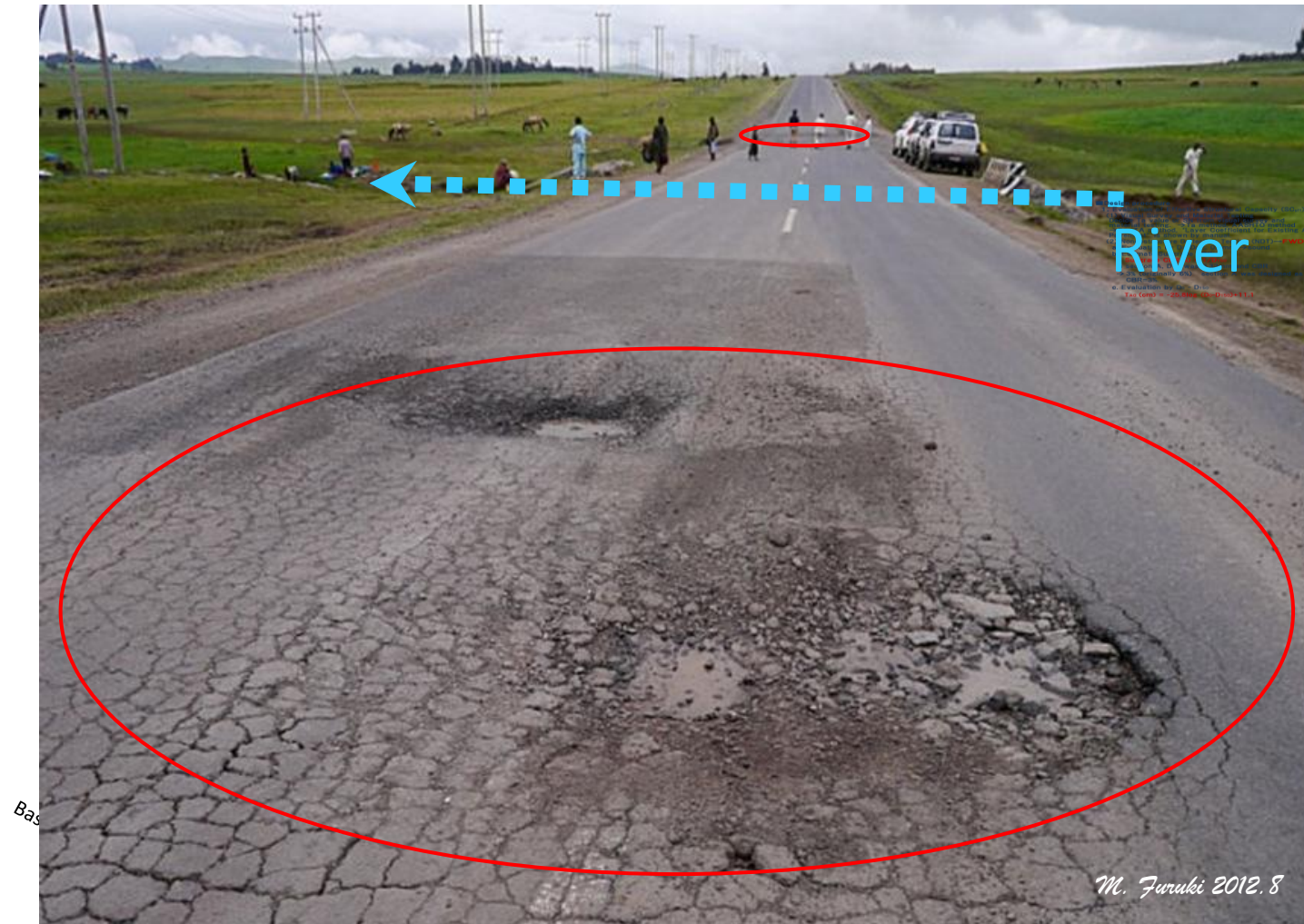
Fig. Damages by water in base course at a sag point. It is symmetrically damaged across the river.
