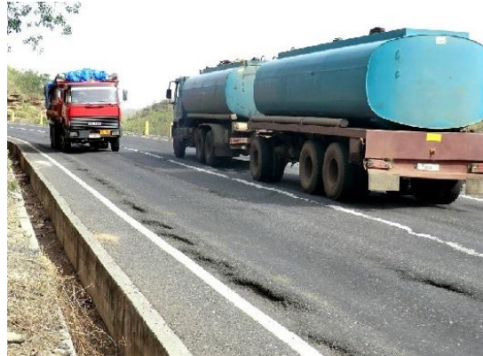
Rutting developed on the steep slope in very hot climate.
