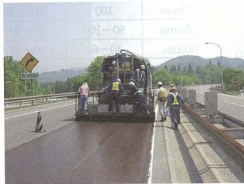
Photograph-4.2.17: Implementation of micro surfacing
