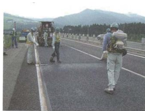
Photograph-4.2.20: Implementation of drainage topcoat
