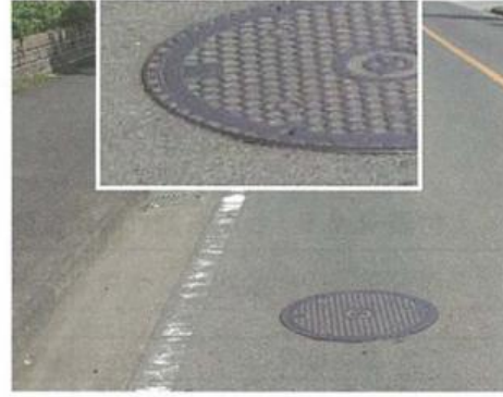
Faulting at a utility hole
