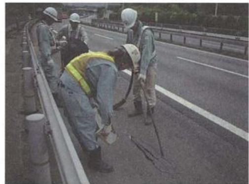
Photograph-4.2.10: Injection of sealant
