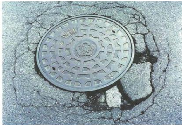
Appendix Photograph-4.2.12: Cracking around structures
