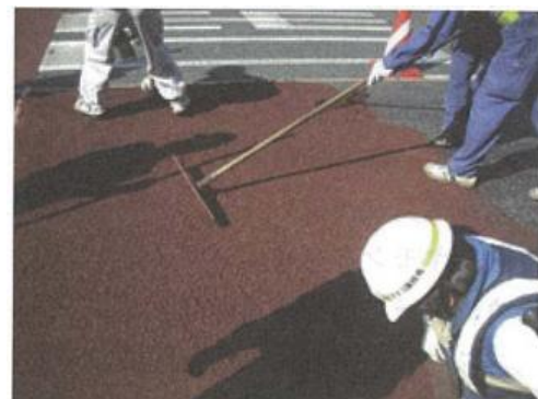
Photograph-4.2.21: Rubbing of permeable resin mortar
