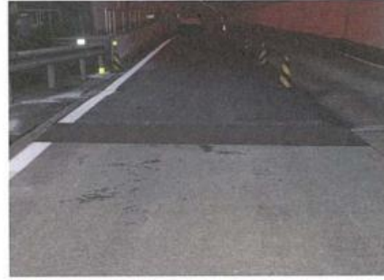
Photograph-4.2.6: Portion whose faulting has been repaired
