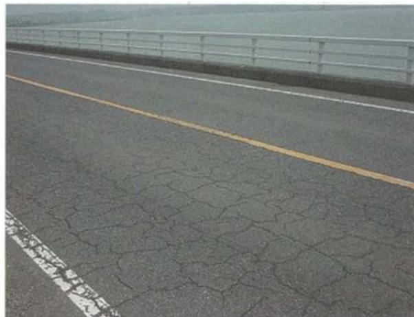
Appendix Photograph-4.2.10: Cracking due to degradation or aging of asphalt
