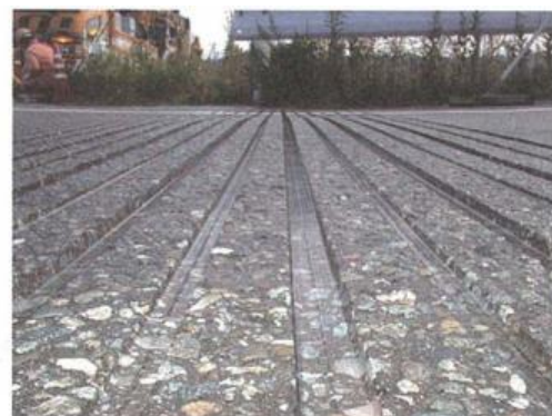
Photograph-4.2.27: Road surface that has undergone grooving
