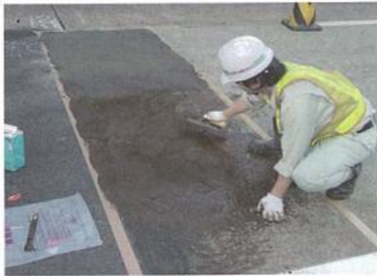
Photograph-4.2.5: Spreading to even a faulting portion
