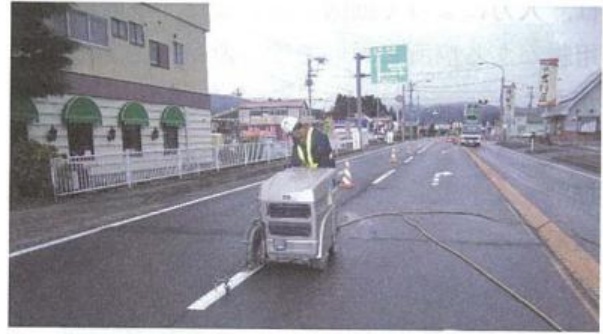
Photograph-4.3.1: Cutting of pavement
