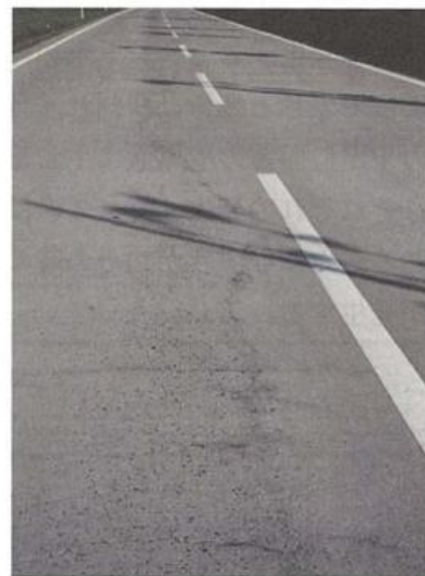
(b) Continuously reinforced concrete pavement
