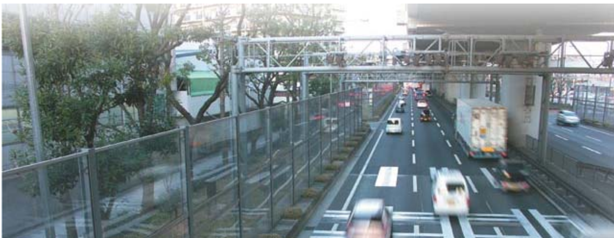
Appendix Photograph-9.4.2: Installed automatic special-vehicle measurement system 4)
