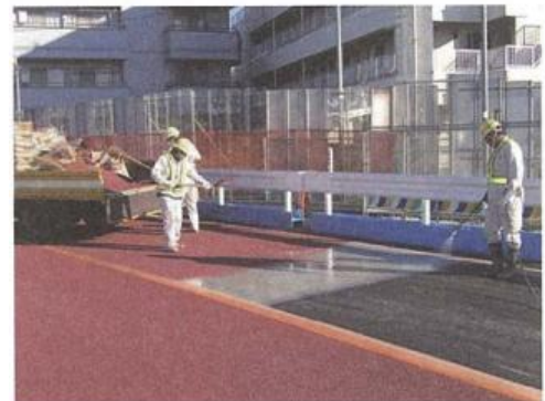
Photograph-4.2.19: Application of resin material
