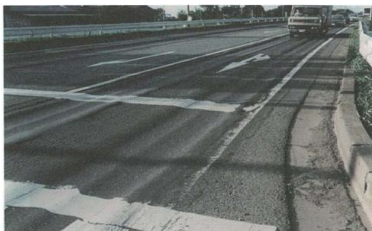
Appendix Photograph-4.2.14: Rutting due to plastic deformation of asphalt mixture
