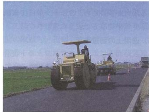
Photograph-4.3.16: Overlay (by rolling)
