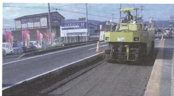
Photograph-4.3.7: Construction of base course (by rolling)
