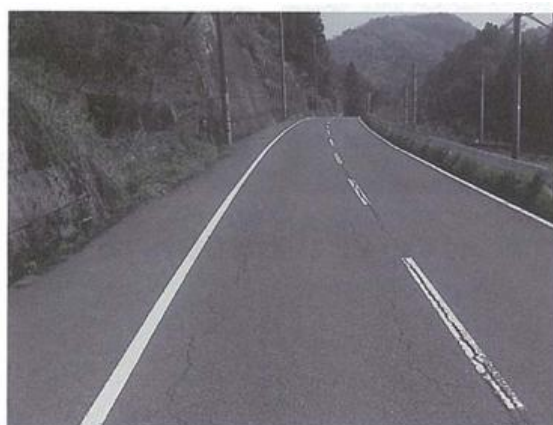
Appendix Photograph-4.2.1: Fatigue cracking
