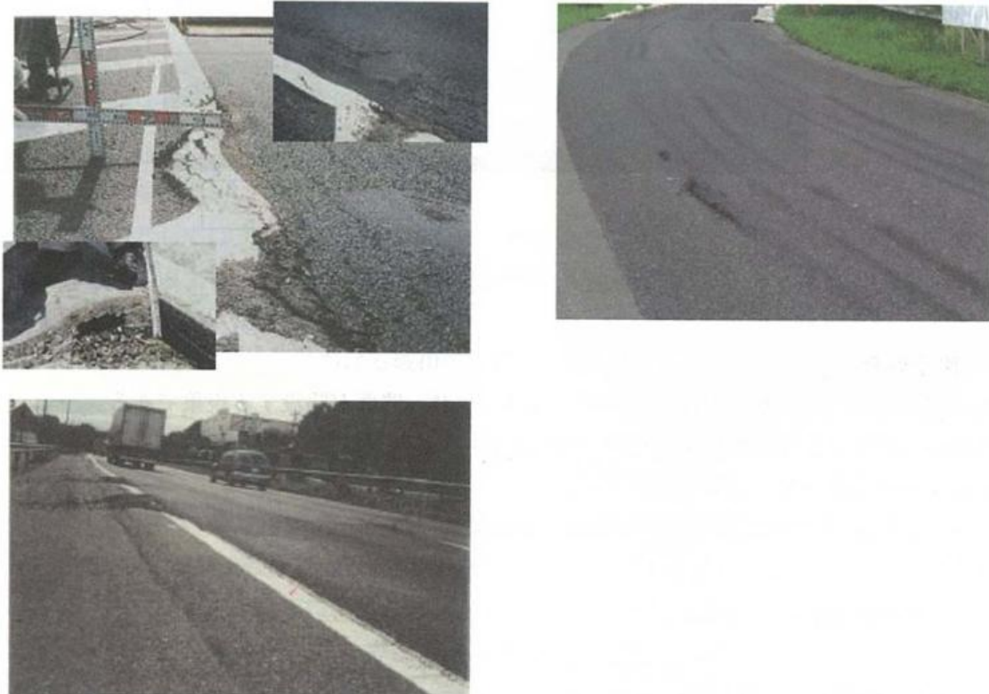
Appendix Photograph-4.2.26: Partial bumps in porous asphalt pavement
