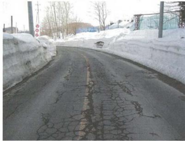
Appendix Photograph-4.2.11: Cracking due to decreased bearing capacity of subgrade or base course during thawing
