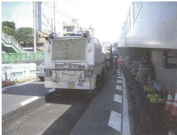
Photograph-4.3.2: Demolition of pavement (by road cutter)
