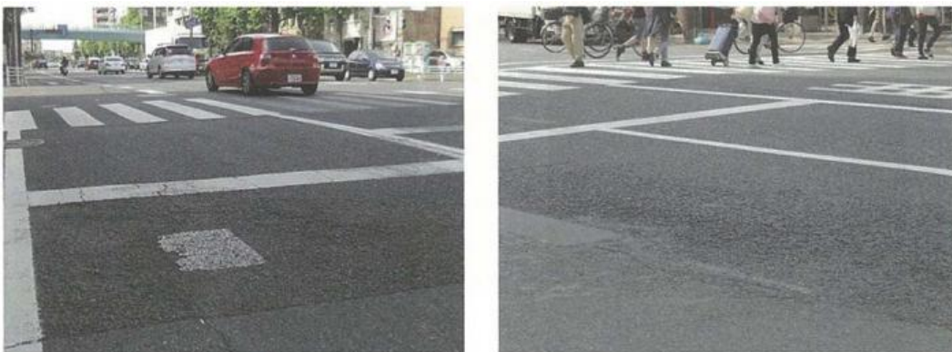
Appendix Photograph-4.2.23: Scattering of aggregate of porous asphalt pavement
