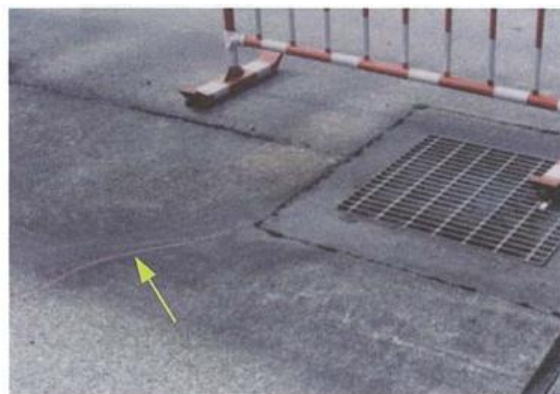
Appendix Photograph-5.2.10: Irregular (restricted) cracking of a concrete pavement slab
