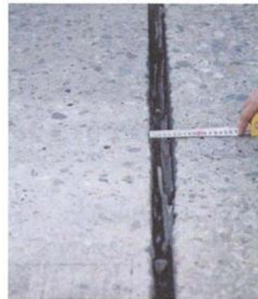
Appendix Photograph-5.2.13: Scattering of joint filler
