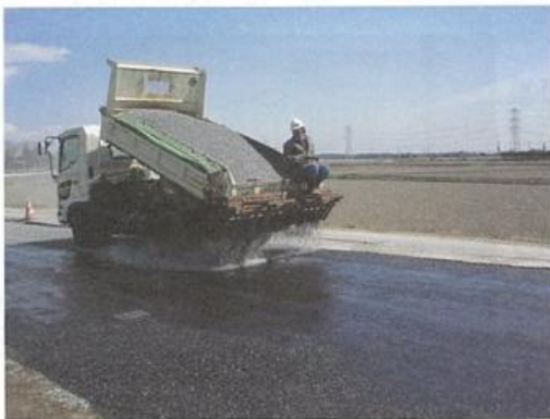
Photograph-4.2.15: Chip seal work
