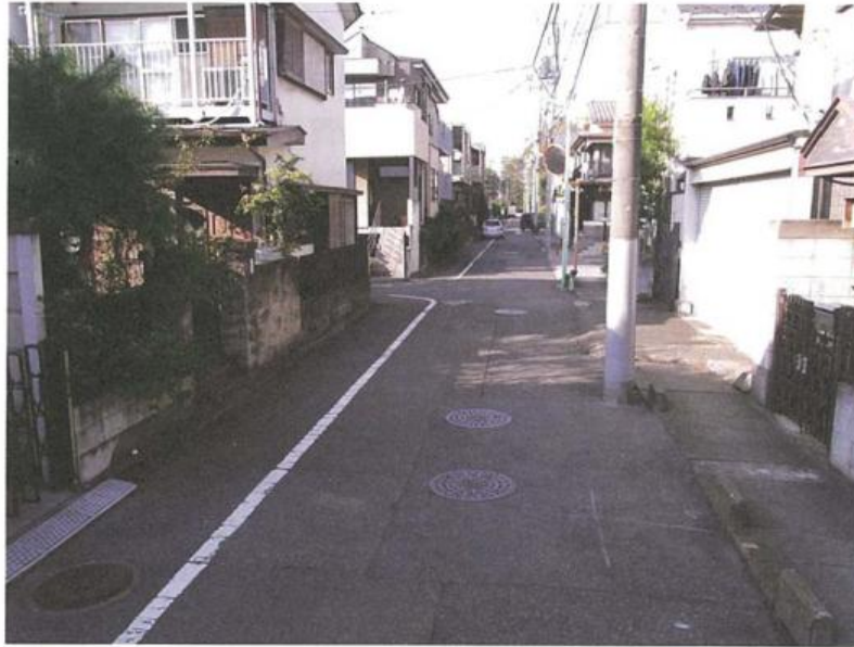
Appendix Photograph-3.2.1: Typical road surface of a daily service road (pavement portions multiple overlap due to recovery)
