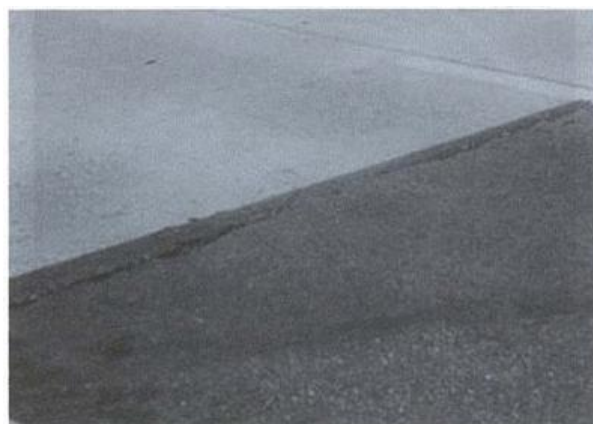
Appendix Photograph-5.2.17: Faulting formed at a joint between a concrete pavement slab and asphalt pavement
