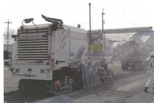
Photograph-4.2.13: Cutting with a road cutter
