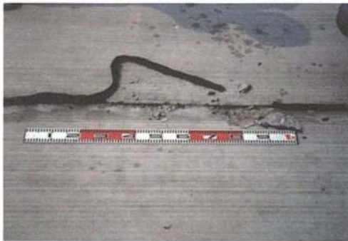
Appendix Photograph-5.2.12: Protrusion of joint filler
