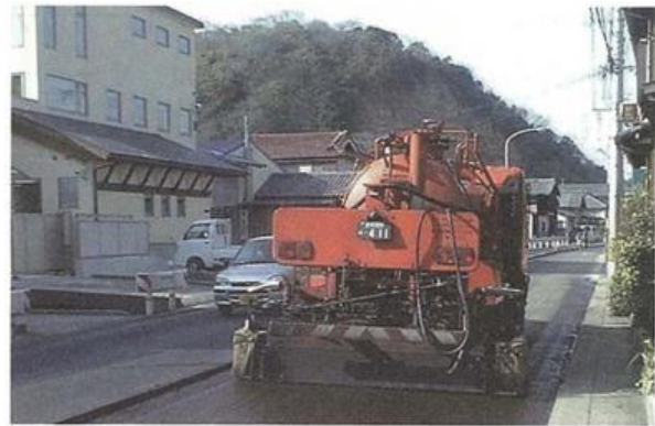
Photograph-4.3.14: Application of tack coat (by distributor)
