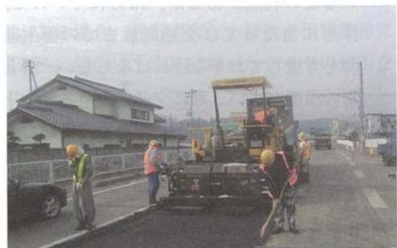
Photograph-4.3.10: Paving (by spreading)
