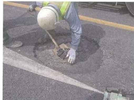
Photograph-4.2.1: Removal of the damage-affected portion
