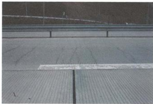
(a) Y-shaped cracking
