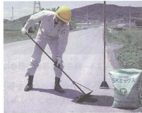
Photograph-4.2.4: Construction using packed material
