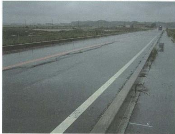
Appendix Photograph-4.2.9: Cracking due to settlement of subgrade or base course
