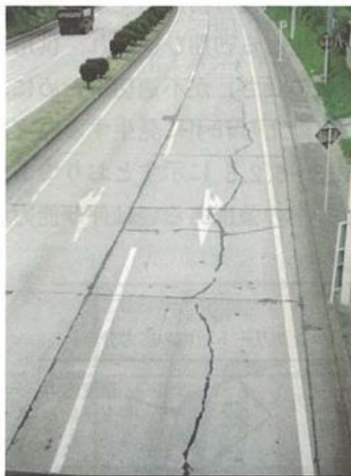
(a) Ordinary concrete pavement
