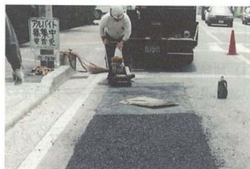
Photograph-4.2.3: Compaction with a blade
