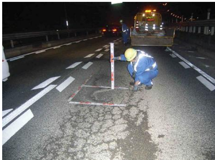
Appendix Photograph-10.2.3: Pavement damaged from confined underground water on a road with canal structure (presented by Metropolitan Expressway Company Limited)
