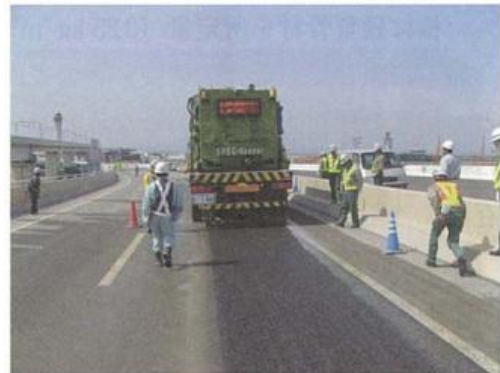
Photograph-4.2.22: Washing of void choking work
