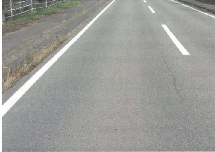
Crack ratio: approx. 5%
