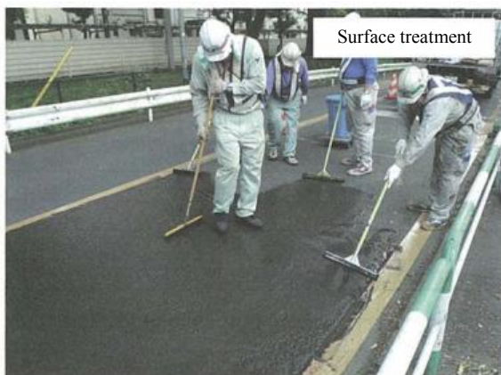
Appendix Photograph-3.5.1: Small-scale surface treatment
