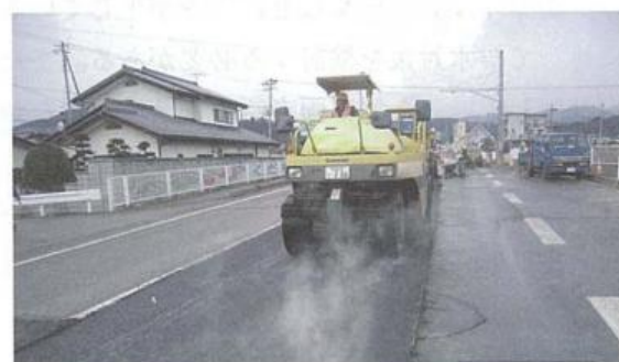
Photograph-4.3.12: Rolling (by pneumatic tire roller)
