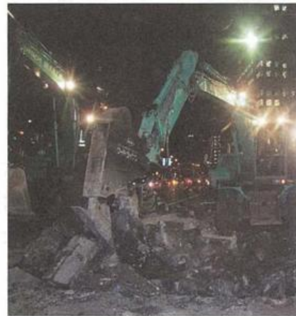
Photograph-4.3.3: Demolition of pavement (by crusher)
