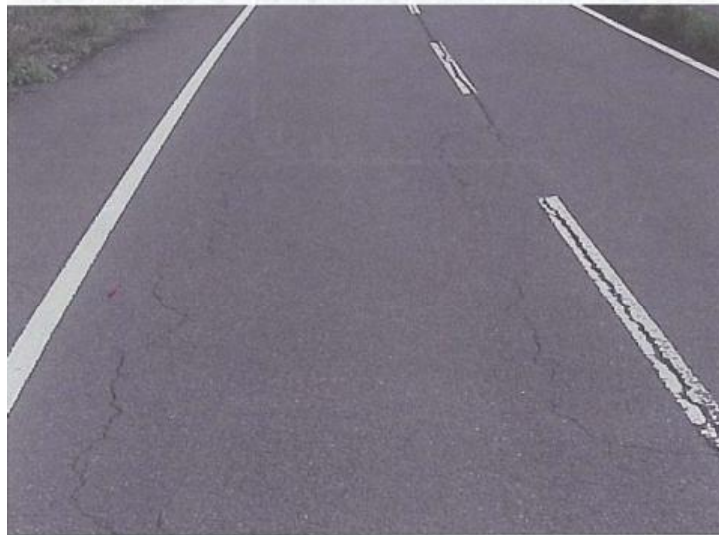
Crack ratio: approx. 20%
