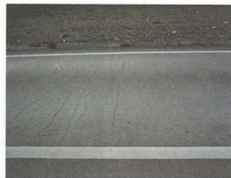
(b) Cluster-type cracking
