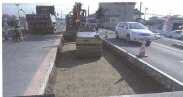
Photograph-4.3.5: Construction of subgrade (by rolling)
