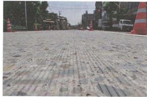
Photograph-4.2.25: Road surface after diamond grinding
