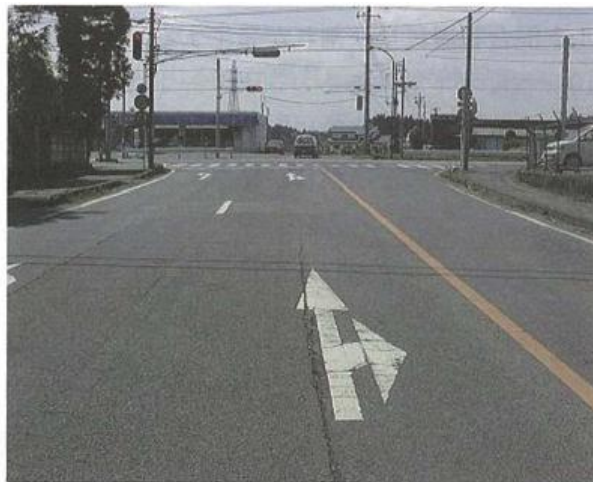
Appendix Photograph-4.2.3: Cracking at a construction joint
