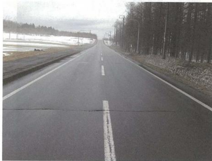
Appendix Photograph-4.2.6: Cracking due to thermal stress
