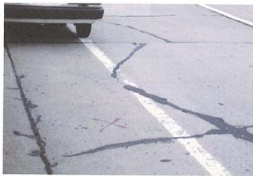
Appendix Photograph-5.2.6: Sheet and alligator cracking of a concrete pavement slab
