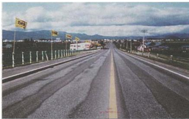
Appendix Photograph-4.2.15: Rutting due to abrasion of asphalt mixture
