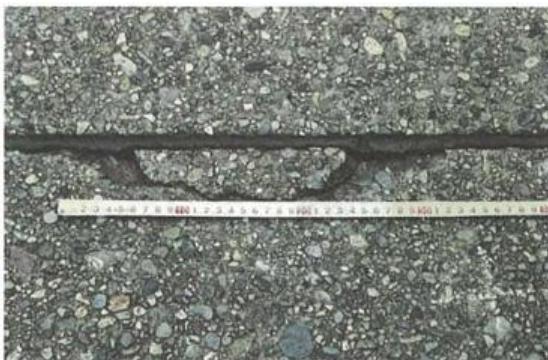
Appendix Photograph-5.2.14: Edge defect at a transverse contraction joint
