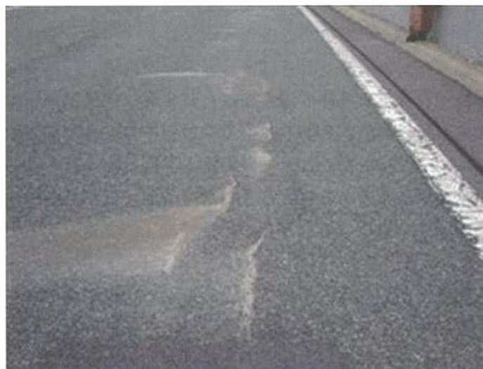
Photograph-3.3.4: Oozing of fine-grained fraction of filler, fine aggregate, etc. onto pavement
