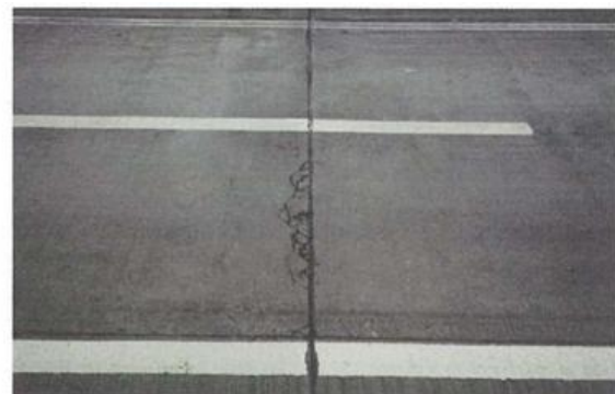
Appendix Photograph-5.2.15: Edge defect at an expansion joint
