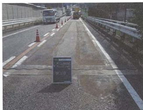
Photograph-4.2.28: Overlay on rutting
