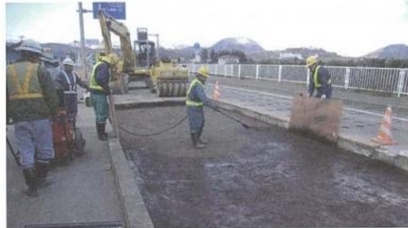
Photograph-4.3.9: Application of emulsion (by sprayer)
