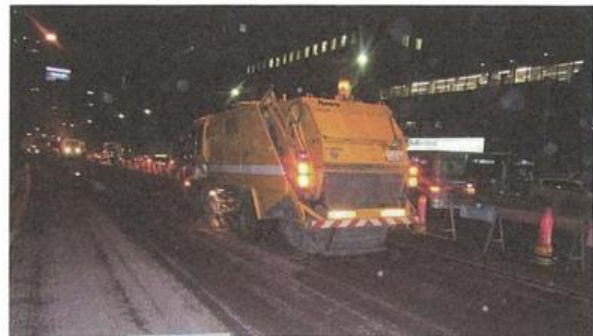
Photograph-4.3.13: Road surface cleaning (by road sweeper)
