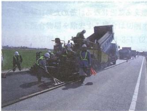
Photograph-4.3.15: Overlay (by spreading)
