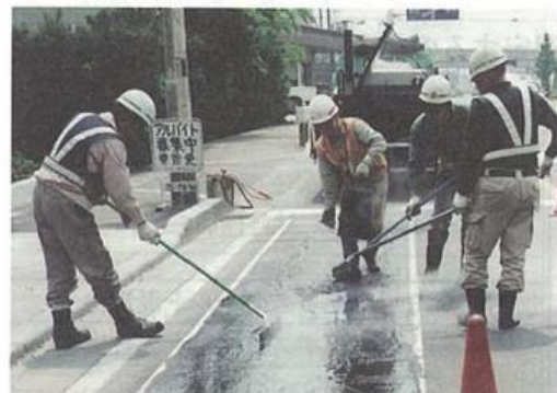
Photograph-4.2.2: Application of special bituminous material
