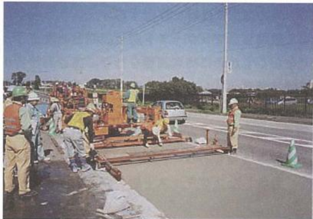
Photograph-4.4.1: Concrete placement
