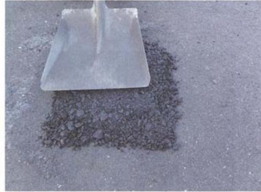
Photograph-4.2.9: Compaction using a shovel back
