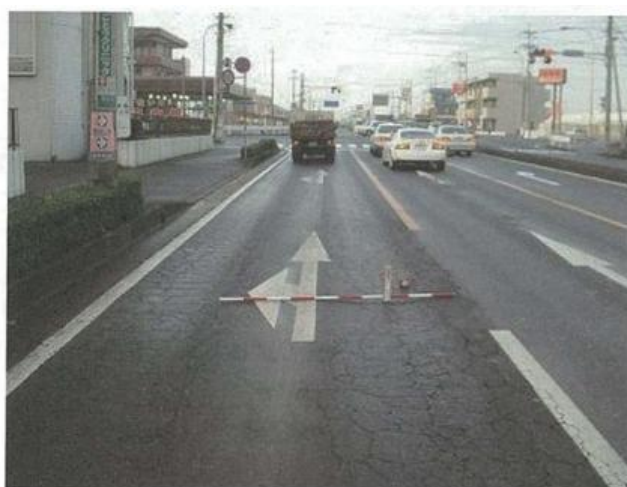
Appendix Photograph-4.2.13: Rutting due to compressive deformation of subgrade or base course
