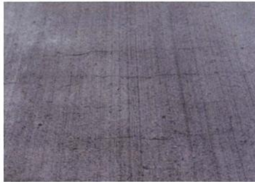
Appendix Photograph-5.2.9: Setting shrinkage cracking of a concrete pavement slab
