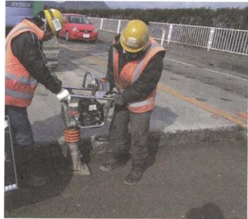
Photograph-4.3.8: Construction of base course (by compaction at edges)
