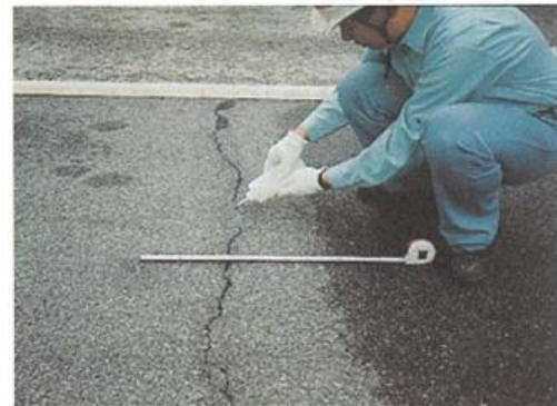
Photograph-4.2.12: Injection of resin-based sealant
