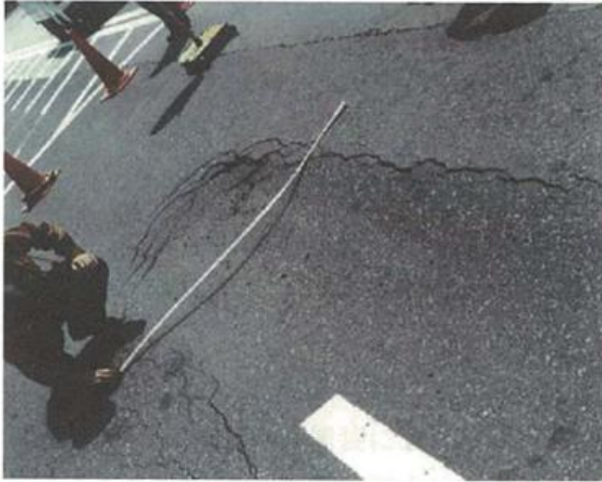
Appendix Photograph-4.2.27: Road surface that is likely to collapse
