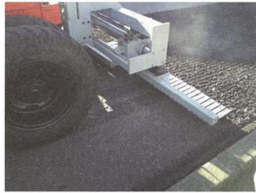
Photograph-4.2.29: Scarification of existing pavement
