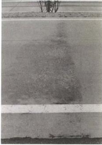
Appendix Photograph-5.2.20: Scaling due to initial frost damage
