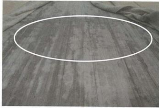
Appendix Photograph-5.2.7: Cracking due to drying of a concrete pavement slab
