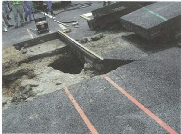
Appendix Photograph-4.2.28: Cavity formed below a road surface
