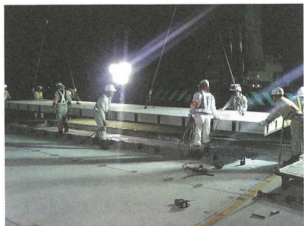
Photograph-4.4.2: Placement of precast concrete slabs
