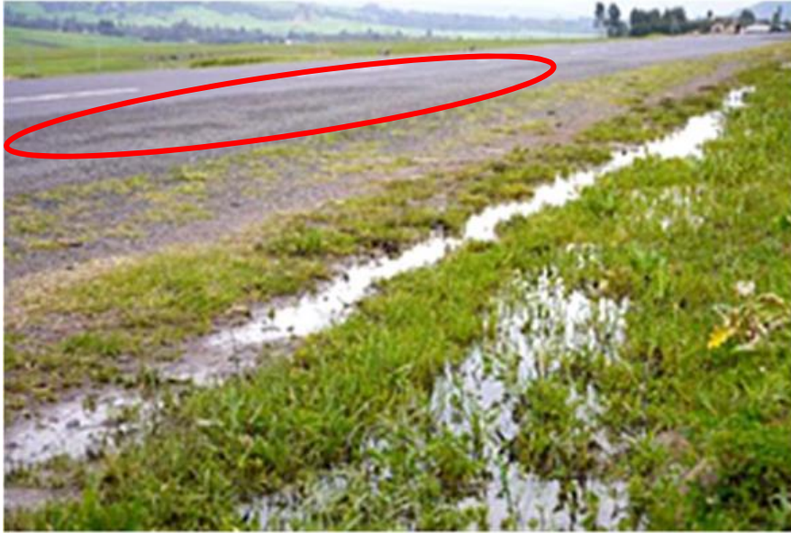
Appendix Photograph-10.2.2: Pavement damaged from underground water from a mountain (earth and sand in the roadside gutter must be excavated.)
