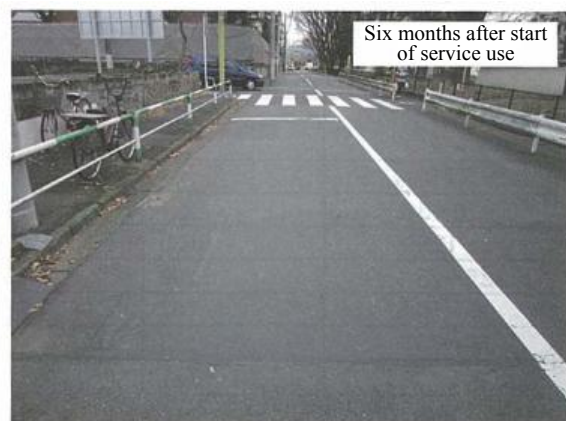
Appendix Photograph-3.5.1: Small-scale surface treatment
