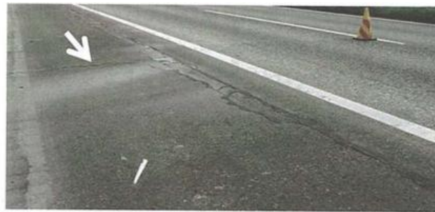
Appendix Photograph-5.2.11: Trace of pumping on a concrete pavement slab
