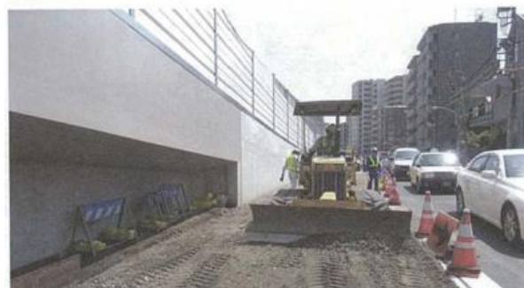
Photograph-4.3.6: Construction of base course (by spreading)
