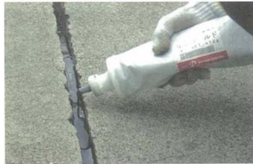
Photograph-4.2.11: Injection of sealant
