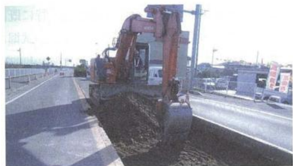
Photograph-4.3.4: Excavation of pavement
