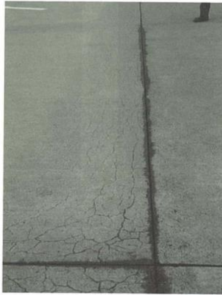
Appendix Photograph-5.2.5: D-cracking of a concrete pavement slab
