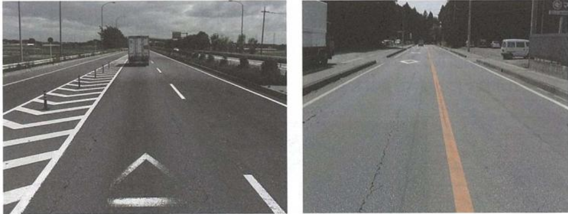
Appendix Photograph-4.2.2: Top-down cracking
