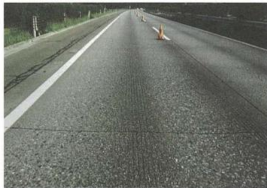
Appendix Photograph-5.2.18: Rutting of a concrete pavement slab
