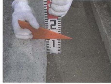
Photograph-5.4.3: Measurement of thickness
