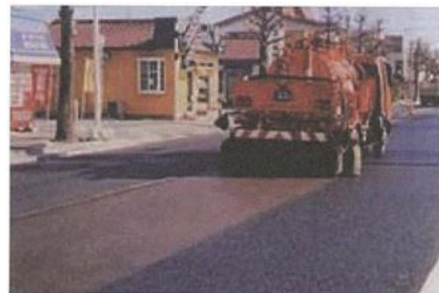
Photograph-4.2.14: Implementation of fog seal
