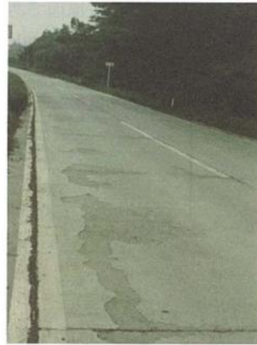
Appendix Photograph-5.2.21: Scaling due to freezing and thawing
