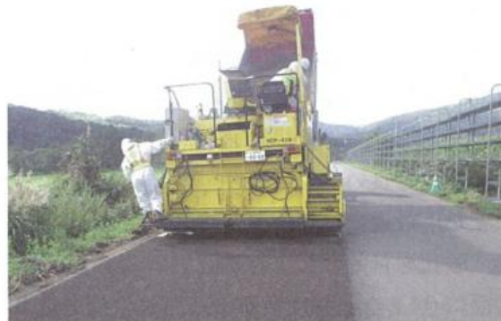
Photograph-4.2.16: Chip seal work using a special machine
