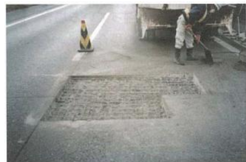
Photograph-4.2.7: Surface after completion of gouging
