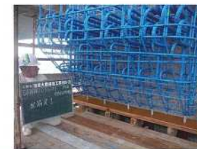
③Reinforcement assembly
