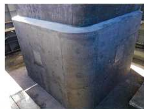
④Wet concrete pouring completed
