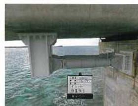
(4) Damper installation completed
