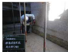
①Reinforcement bar exploration work
