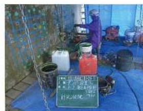
(2) Anchor reinforcement drilling
