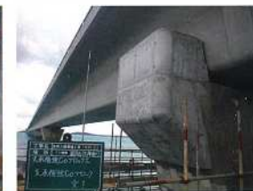
④Bearing reinforcement completed
