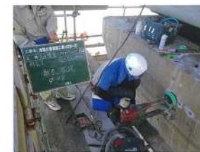
①Hole drilling
