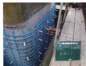
③Reinforcement assembly
