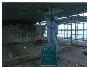
©Reinforcement bar exploration work
