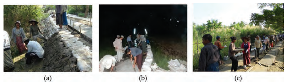
Figure 15. Construction at village K: (a) Covering Do-nou with clay; (b) working at night; (c) bucket brigade for casting concrete.
