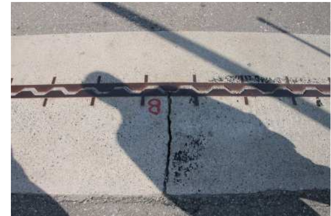
Breakage of expansion device, crack in parapet
