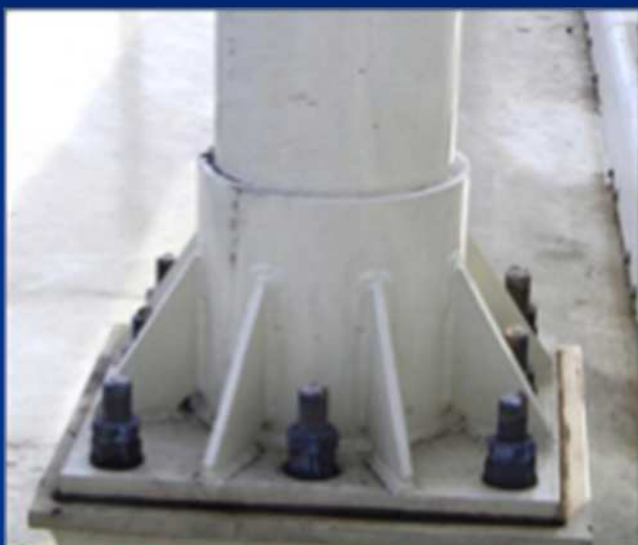
Insulated at base plate
