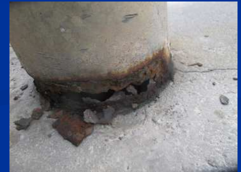
Ring corrosion with through-hole
