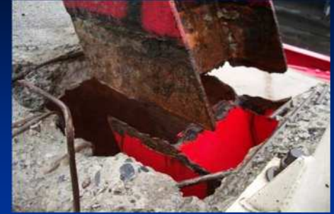
Rupture of truss diagonal member
