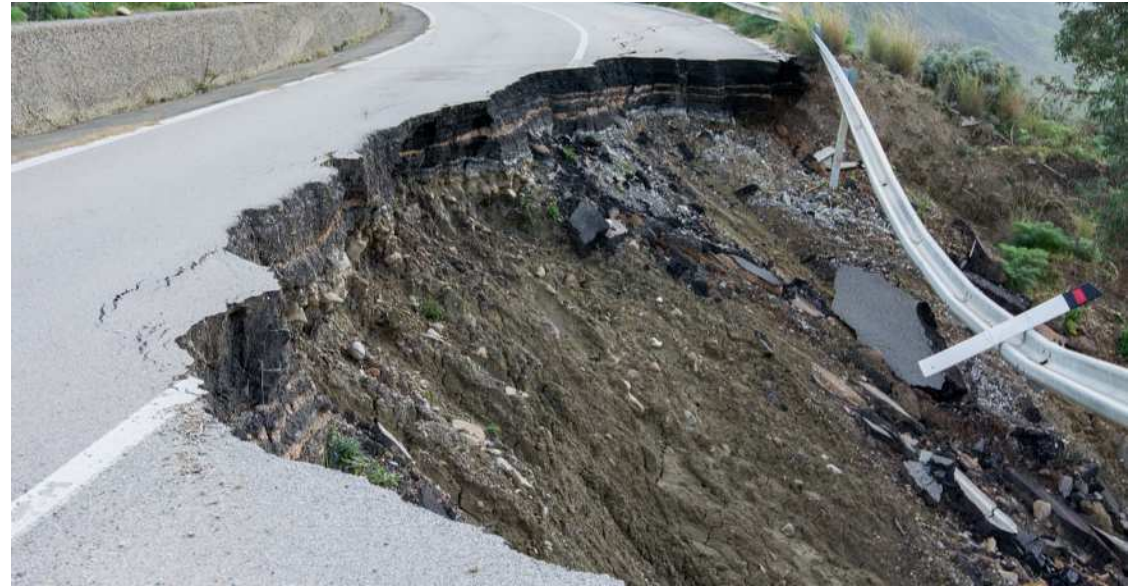
Collapse of road embankment caused by earthquake
