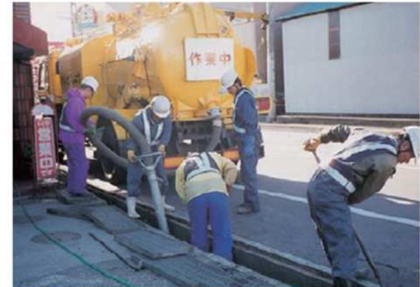
Cleaning roadside ditches with a vacuum truck
