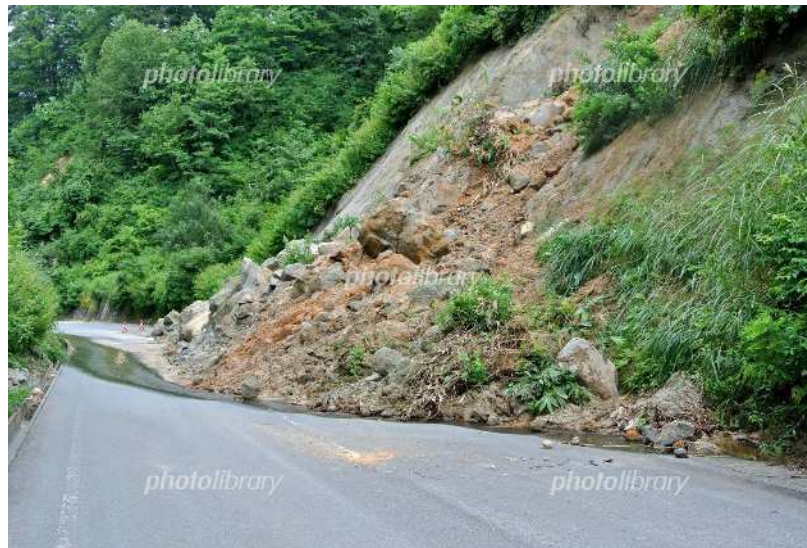
Cliff collapse caused by heavy rain that loosened the ground
