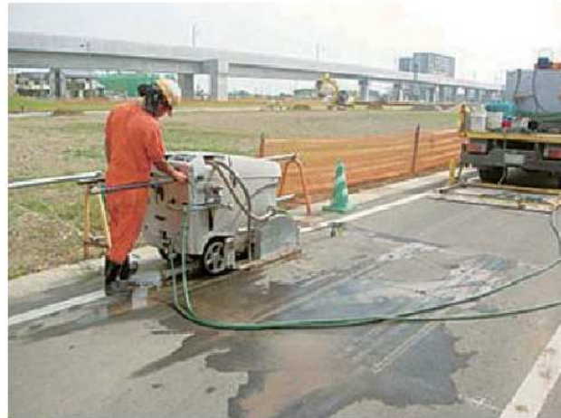
Pavement road cutting work using a concrete cutter
