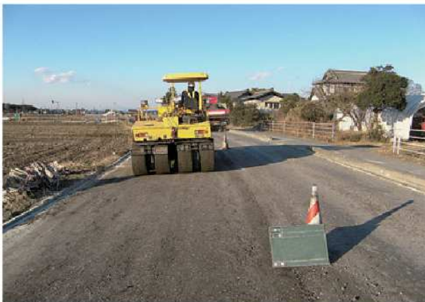
Road base compaction work using tire rollers
