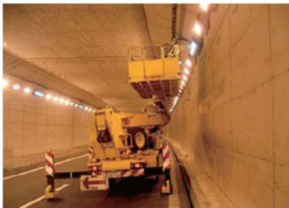
Tunnel lighting cleaning work using elevating vehicles
