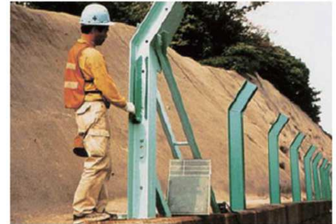
Painting work for rockfall prevention fence posts
