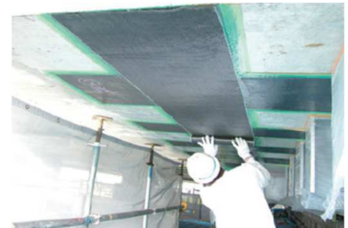
Carbon fiber sheet reinforcement work for concrete floor slabs
