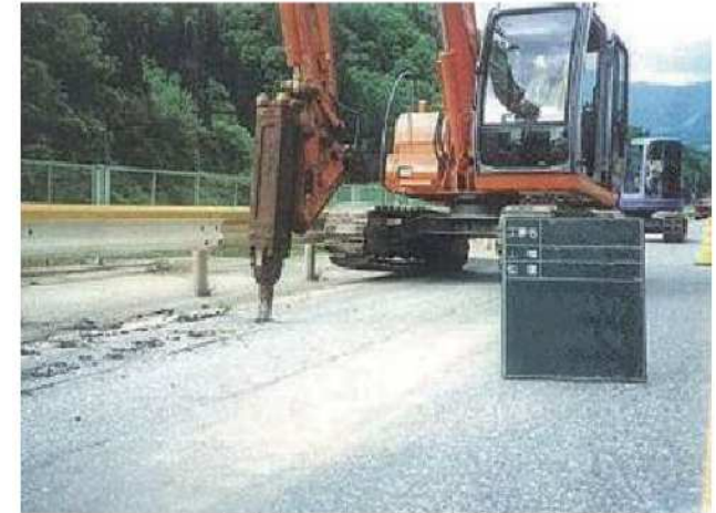
Pavement breaking work using large breakers
