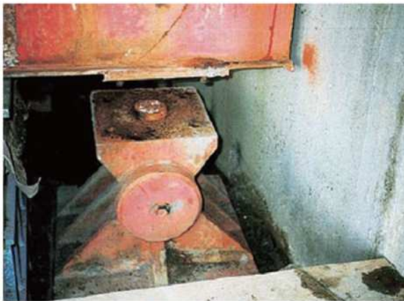
Bridge bearing replacement (old bearing)
