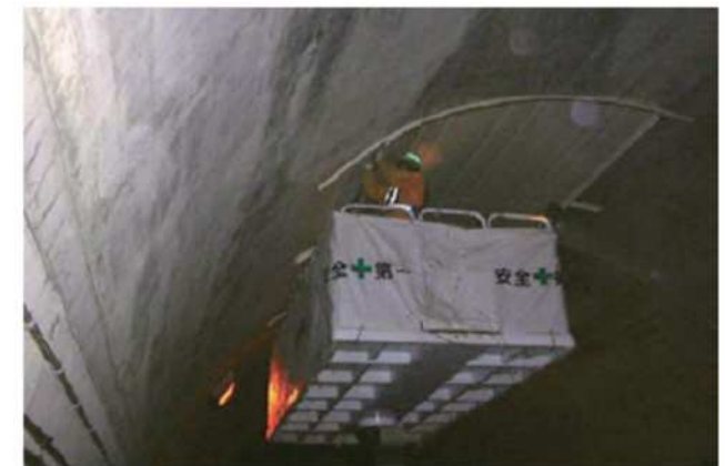
Installation of waterproof board by elevating truck
