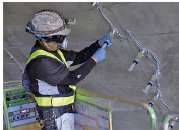
Tunnel lining crack prevention injection work
