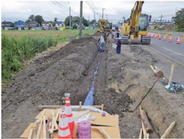
Installation of sheath pipes for electric wires, optical cables, etc.
