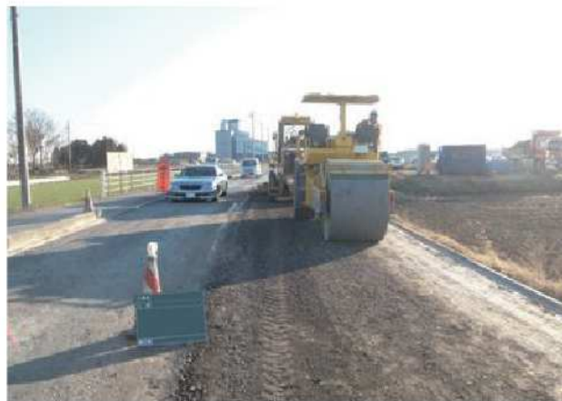
Road base compaction work using road rollers
