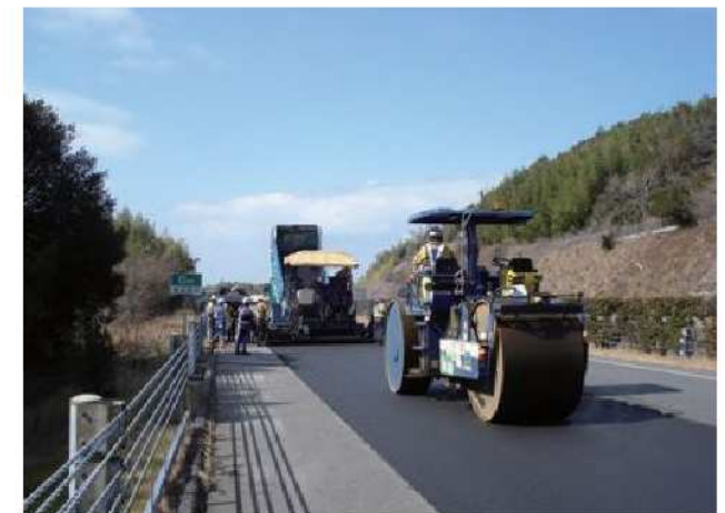
Road compaction work using road rollers
