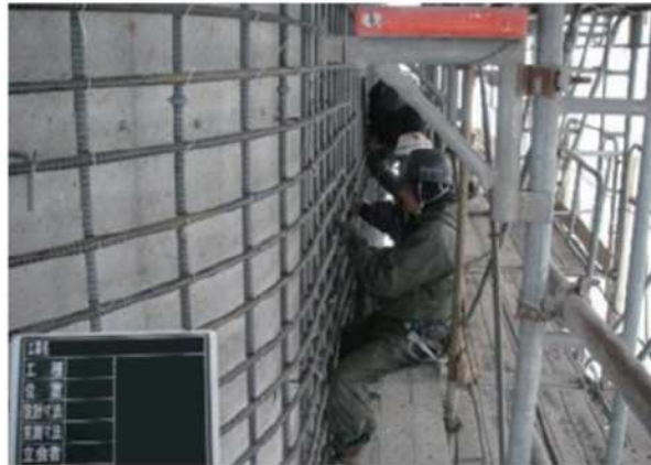
Concrete reinforcement and steel anchor work for bridge piers
