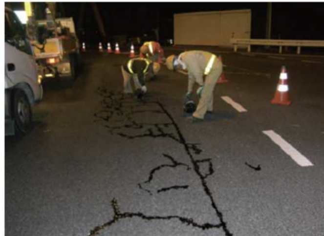
Asphalt melt injection work for pavement cracks
