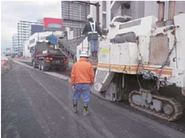
Paved road surface cutting work
