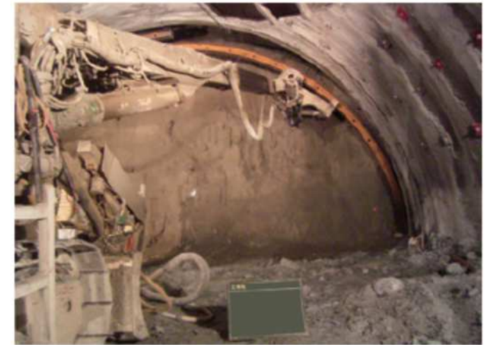
Fig. 7 Steel shoring construction status ④
