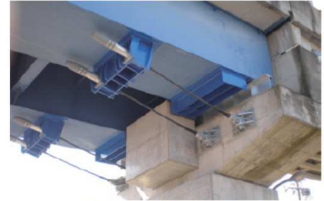
Bridge collapse prevention using PC steel bars on bridge piers
