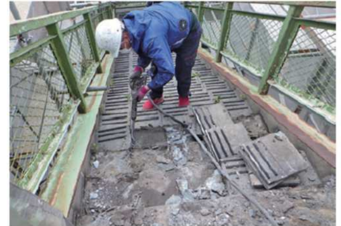
Pedestrian bridge stairs repair work
