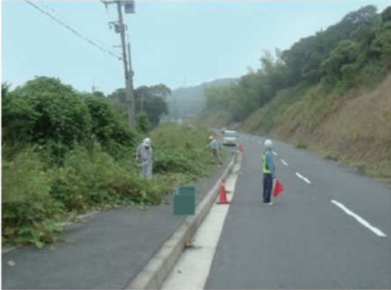
Road weeding with shoulder-mounted mower
