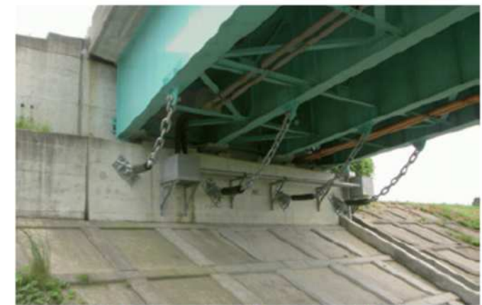
Bridge collapse prevention using bridge pier chains
