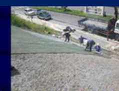
(23) Welded metal net installation
