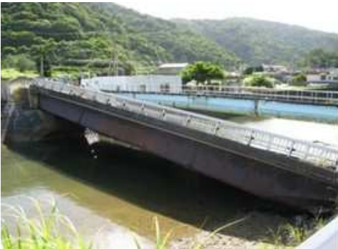
A collapsed bridge by aging
