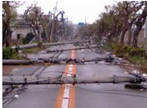
Utility poles collapsed by typhoon
