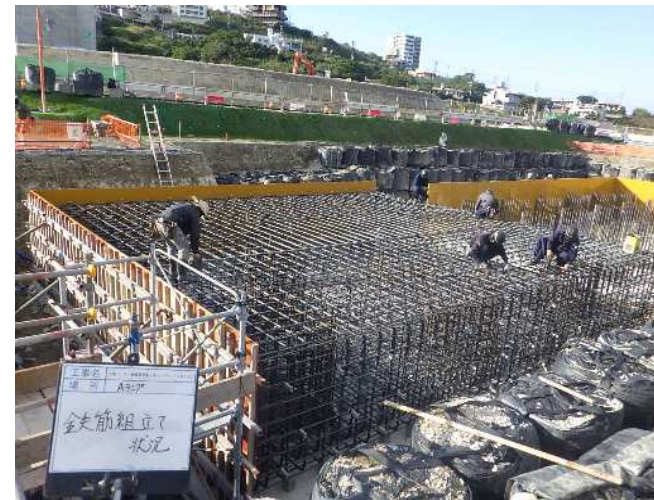
Bottom plate rebar assembly
