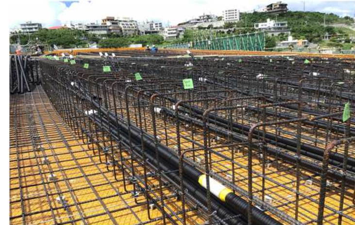
7-5-3 PC cable sheath (overall view)
