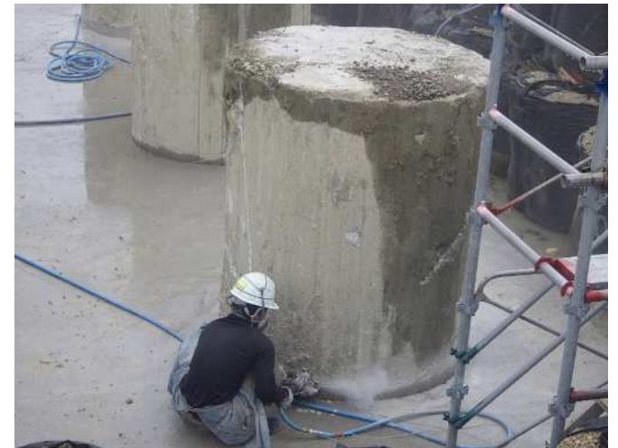
Pile head treatment construction
