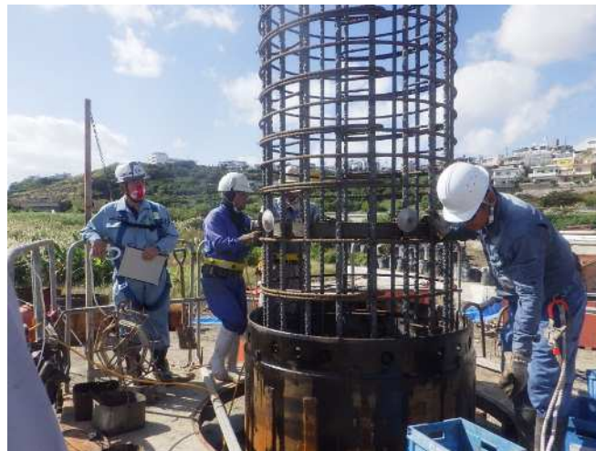
Installing the steel cage and spacers
