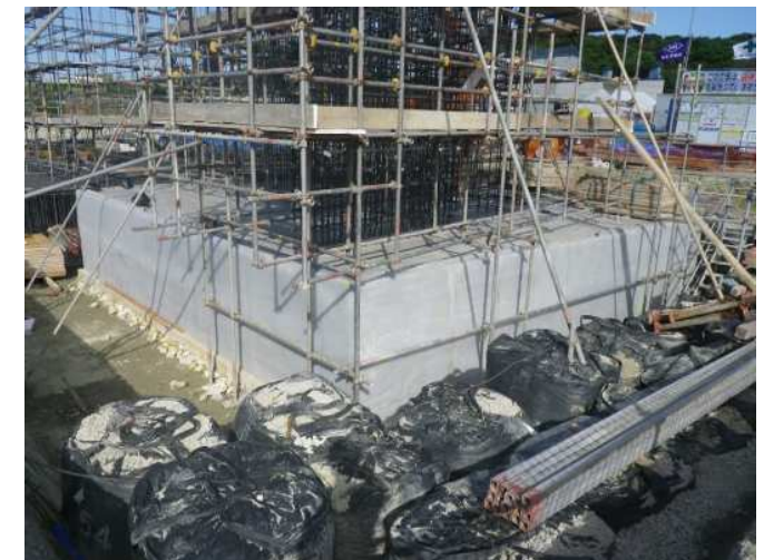
Formwork removal
