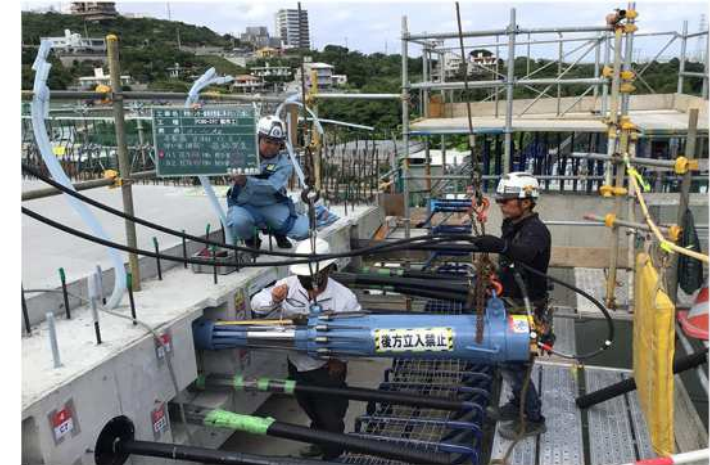
7-5-5 Cable tensioning
