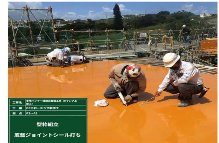
7-5-1 Formwork assembly
