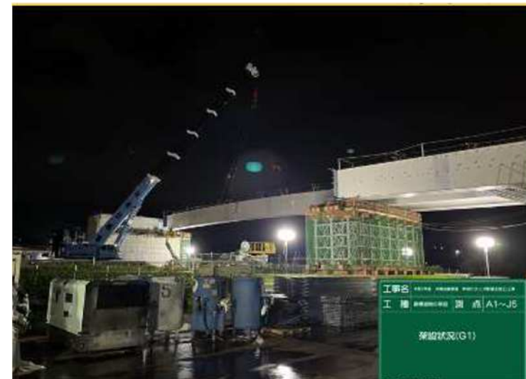
550t lifting crane assembly Large block erection (2B) between A1 and vent
