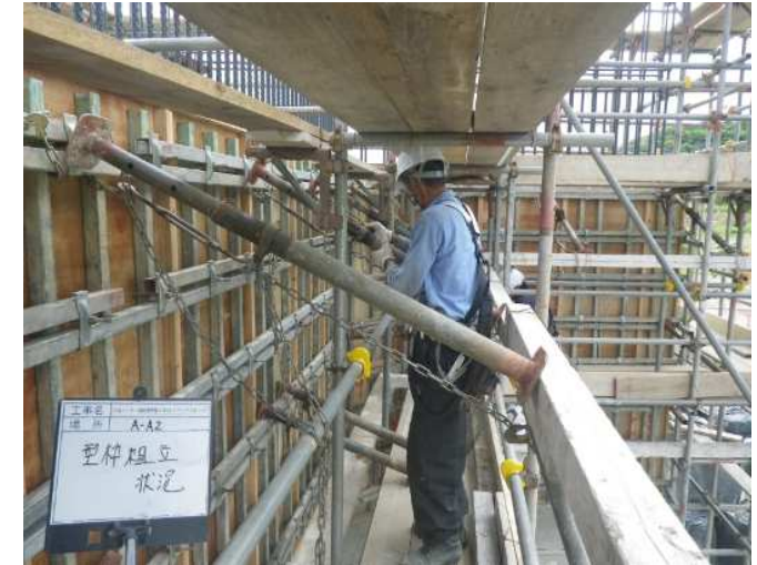
Assembling vertical formwork (1st lot)
