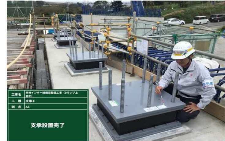
7-3 Rubber bearing construction
