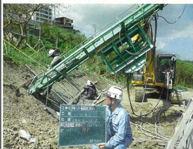
1-3 削孔角度確認・削孔
