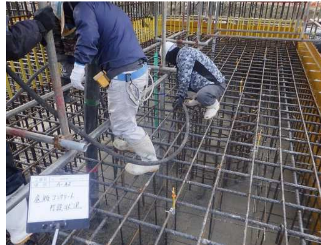
Pouring concrete for base plate
