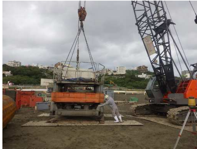
Excavation machine installation (full rotary machine installation)
