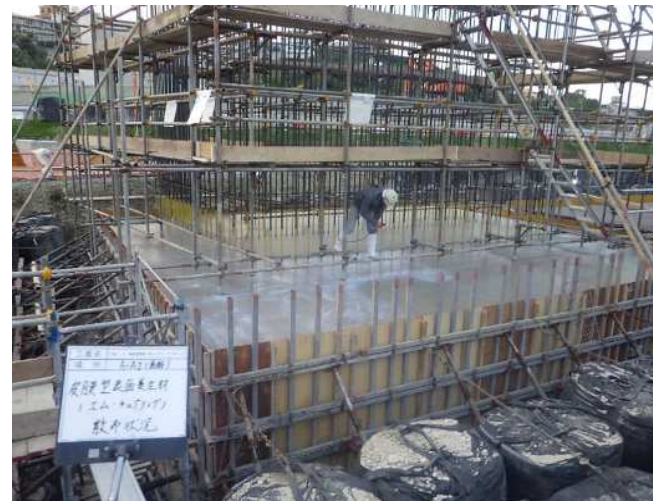
Pouring of base concrete completed
