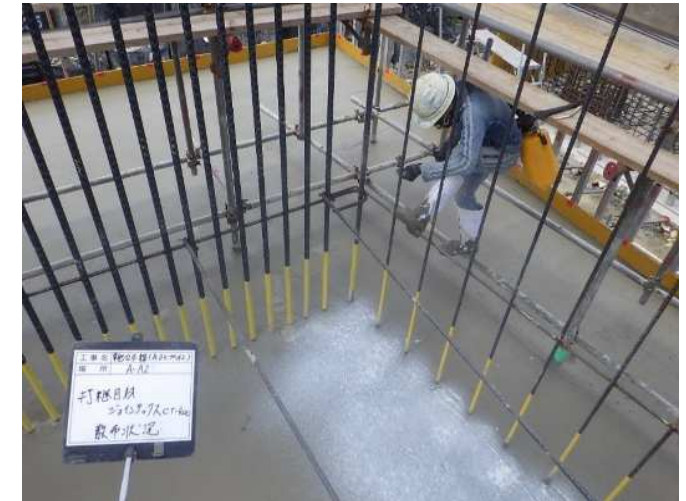
Spreading concrete curing material
