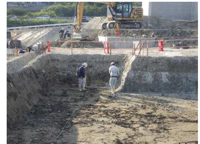
Magnetic exploration (stratigraphic exploration)
