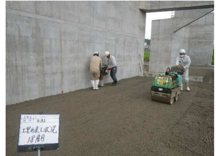
Backfilling
