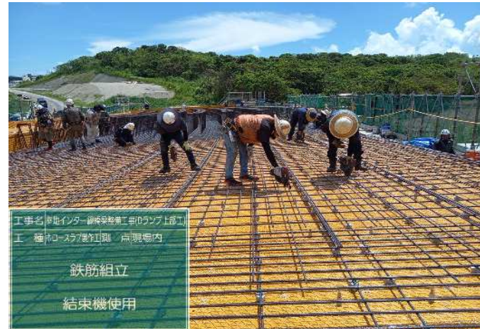
7-5-2 Reinforcing bar assembly (lower bar)
