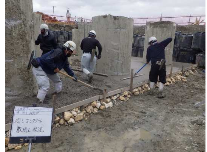
Pouring smooth concrete
