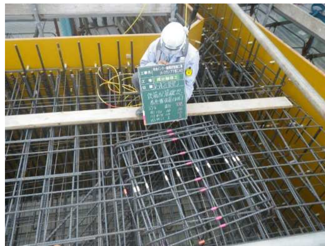
Vertical wall rebar assembly (3rd lot)
