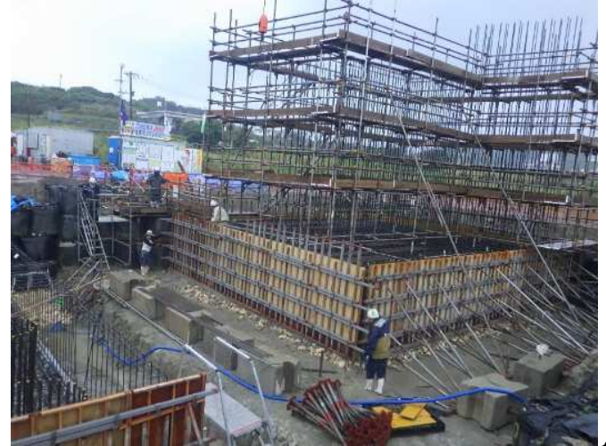
Bottom slab formwork assembly
