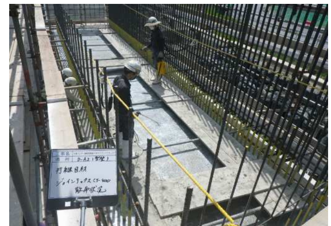
Spraying treatment material for vertical wall concrete joints
