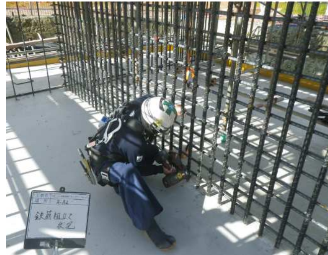
Assembling vertical wall rebar (1st lot)
