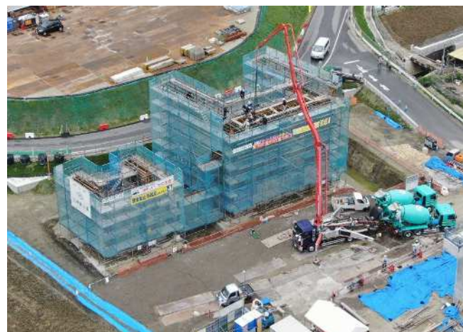
Pouring concrete for vertical walls (3rd lot)
