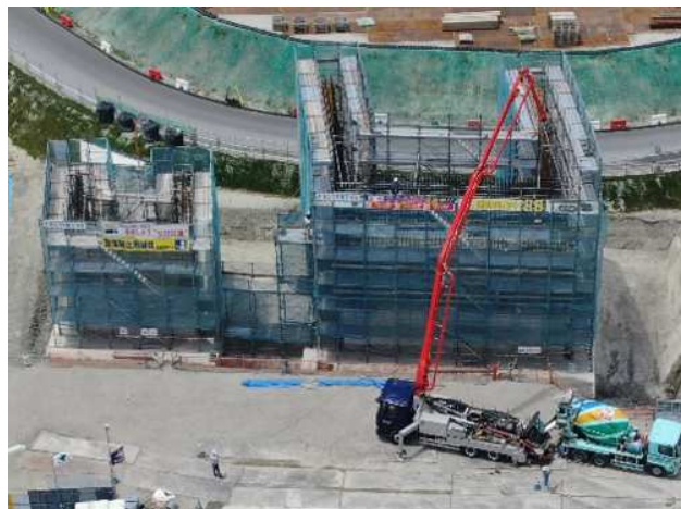
Pouring concrete for vertical walls (2nd lot)
