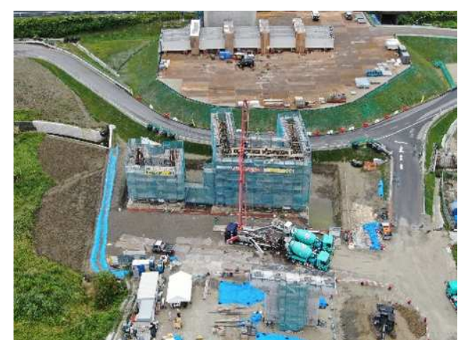
Vertical wall concrete pouring (3rd lot)
