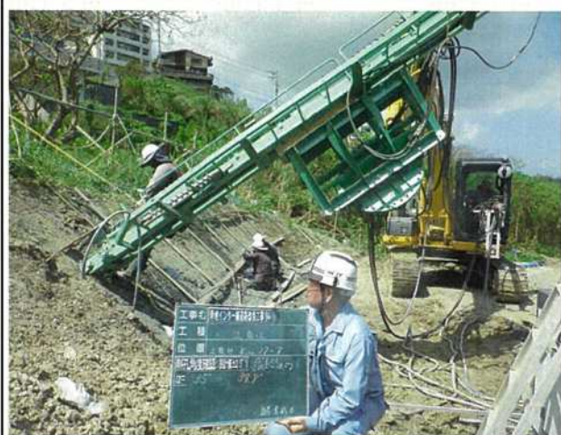
1-3 削孔角度確認・削孔
