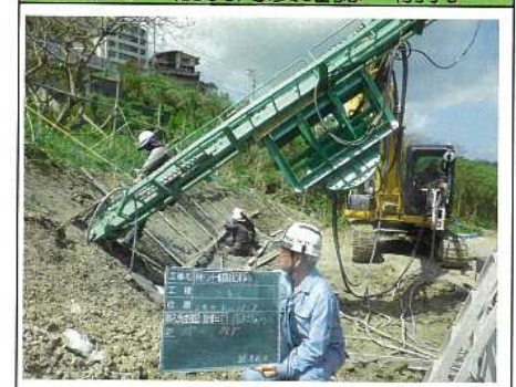
1-3 削孔角度確認・削孔
