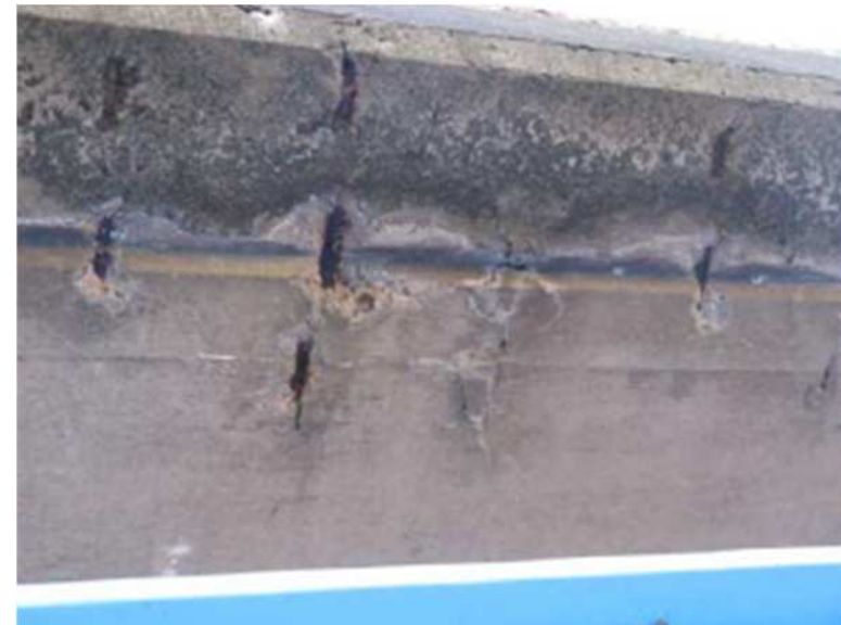
Rebar exposure due to insufficient coverage
