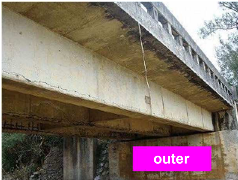
Example of the difference in damage between outer and inner surfaces of an outer girder
