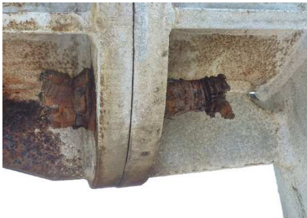
Bolt and nut breakage
