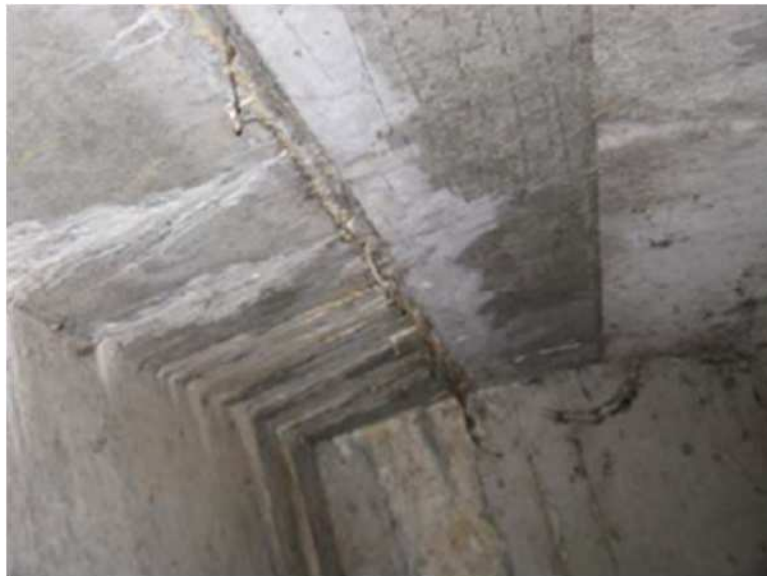
Free lime spillage/leakage from bed slab joints
