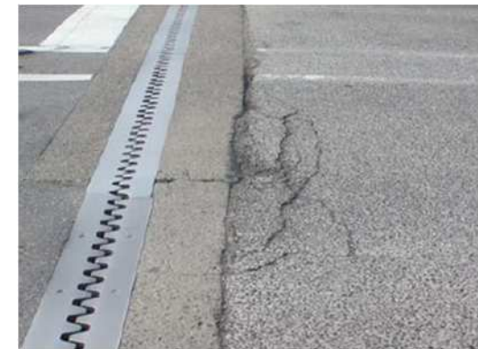
Example of pavement cracks on back of abutment
