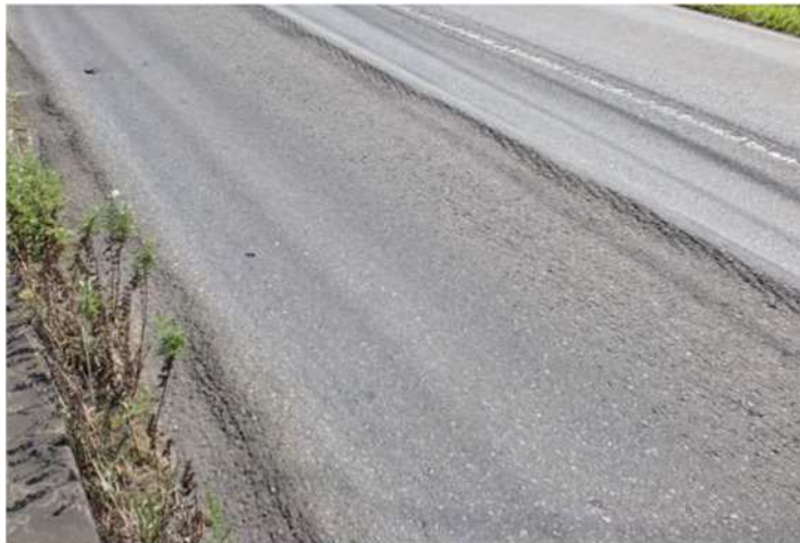
Example of rutting caused by compressive deformation of roadbed/subgrade
