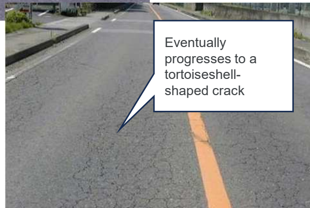
Example of cracks (final stage)
