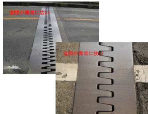
Examples of anomalies in expansion devices
