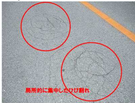
Examples of cracks on pavement surfaces
