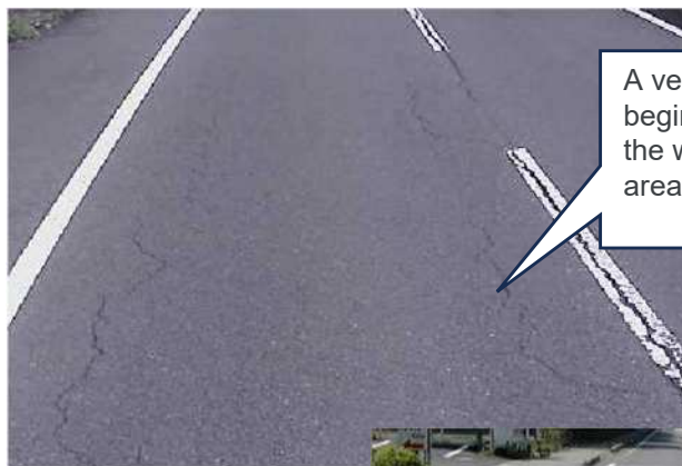
Example of cracks (early stage)
