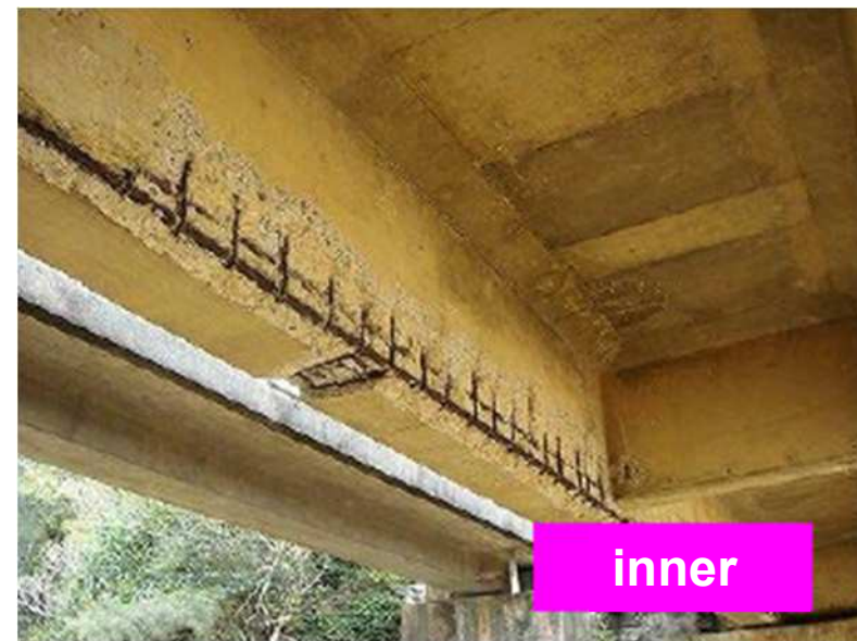
Example of the difference in damage between outer and inner surfaces of an outer girder
