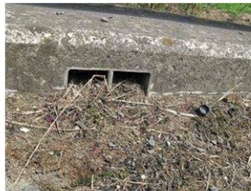
Example of sediment clogging in drainage basin
