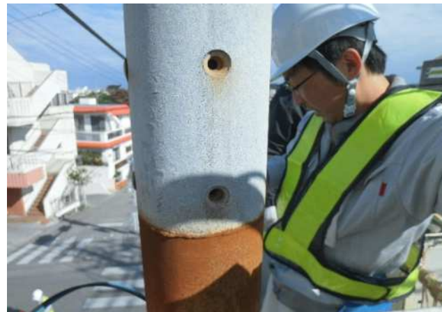
Bolt detachment at the pillar joint
