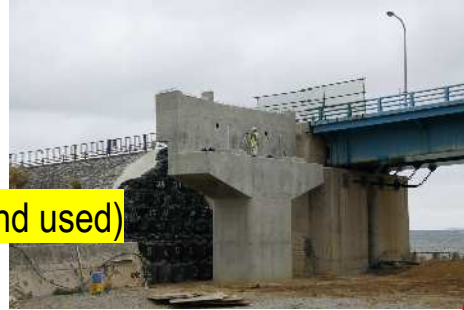
New Motobu Bridge (Substructure: C- & S-replaces)
