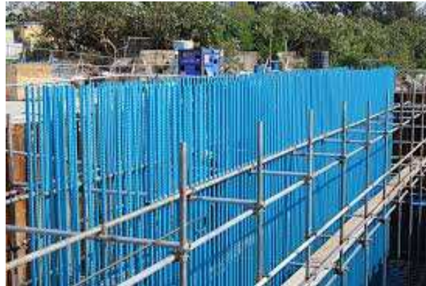
Epoxy resin coated rebar
