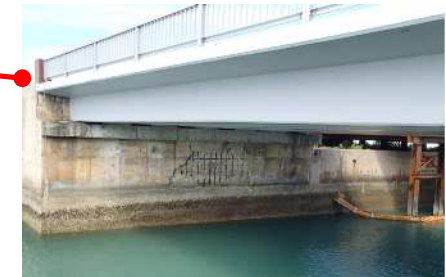
Awase Bridge (tentative name) (Superstructure: S-replace, substructure: C- & S-replaces)
