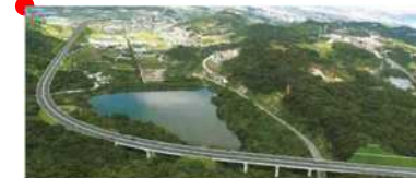
Awase Bridge (tentative name) (Superstructure: S-replace, substructure: C- & S-replaces)
