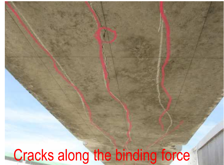
When the internal binding force is large
