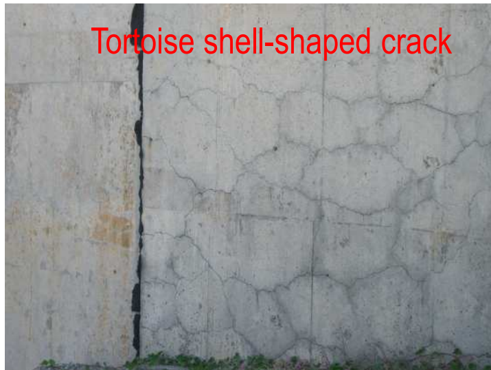
When the internal binding force is small
