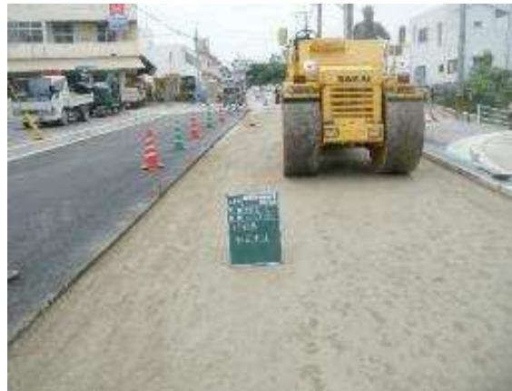
Roadbed materials Paving work
