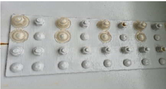
Bolt cap to counter corrosion
